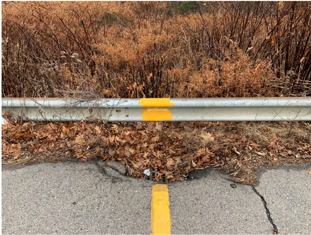
Photo 11 - Catch basin at the edge of pavement on the downstream side of the crest (opposite the catch basin shown in Photo 10). This catch basin discharges into an 18-inch diameter corrugated metal outfall pipe that daylights through the toe of the downstream slope (see Photo 16).
