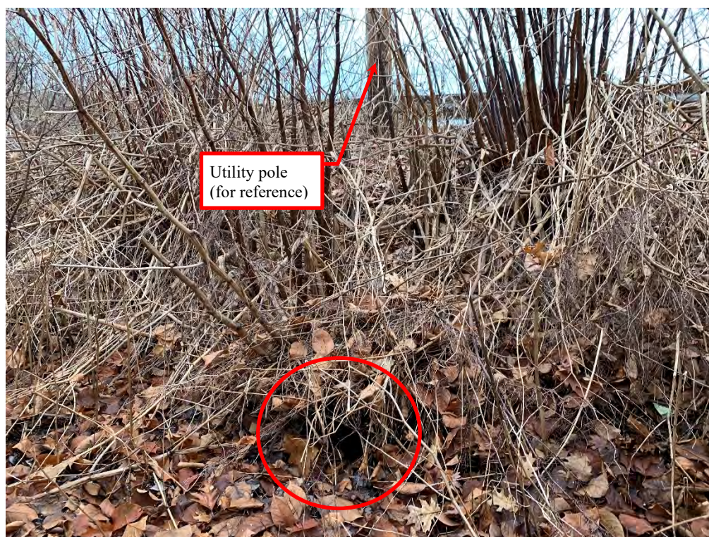
Photo 16 - The partially buried outfall of an 18-inch corrugated metal stormwater drain pipe connected to a catch basin on the dam crest. This outfall is located on the downstream slope between the spillway and left abutment.
