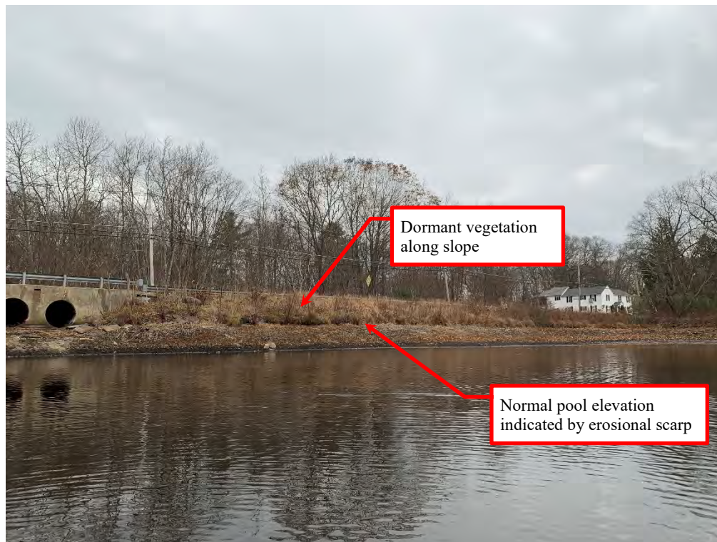
Photo 3 - Overview of the upstream slope (right of the spillway). Note the presence of dormant brush and saplings on the upper portion of the slope above the normal pool elevation.
