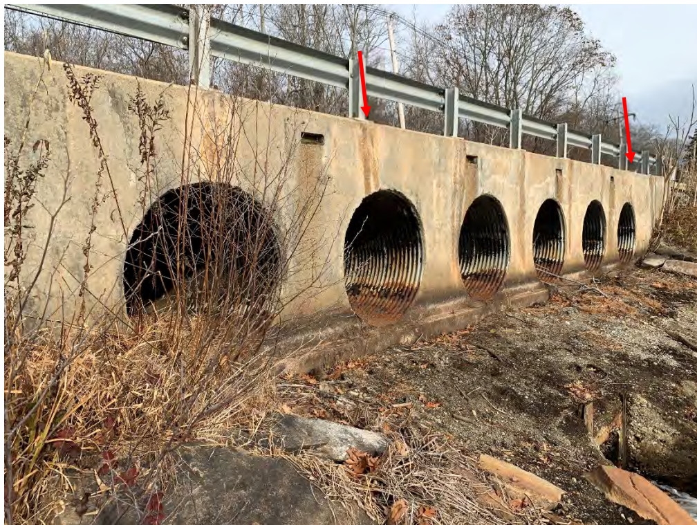
Photo 18 - Overview of the spillway and reinforced concrete headwall. Transverse cracks were observed above the second and sixth CMPs from the left and a longitudinal crack was observed between the third and fourth CMPs from the left.
