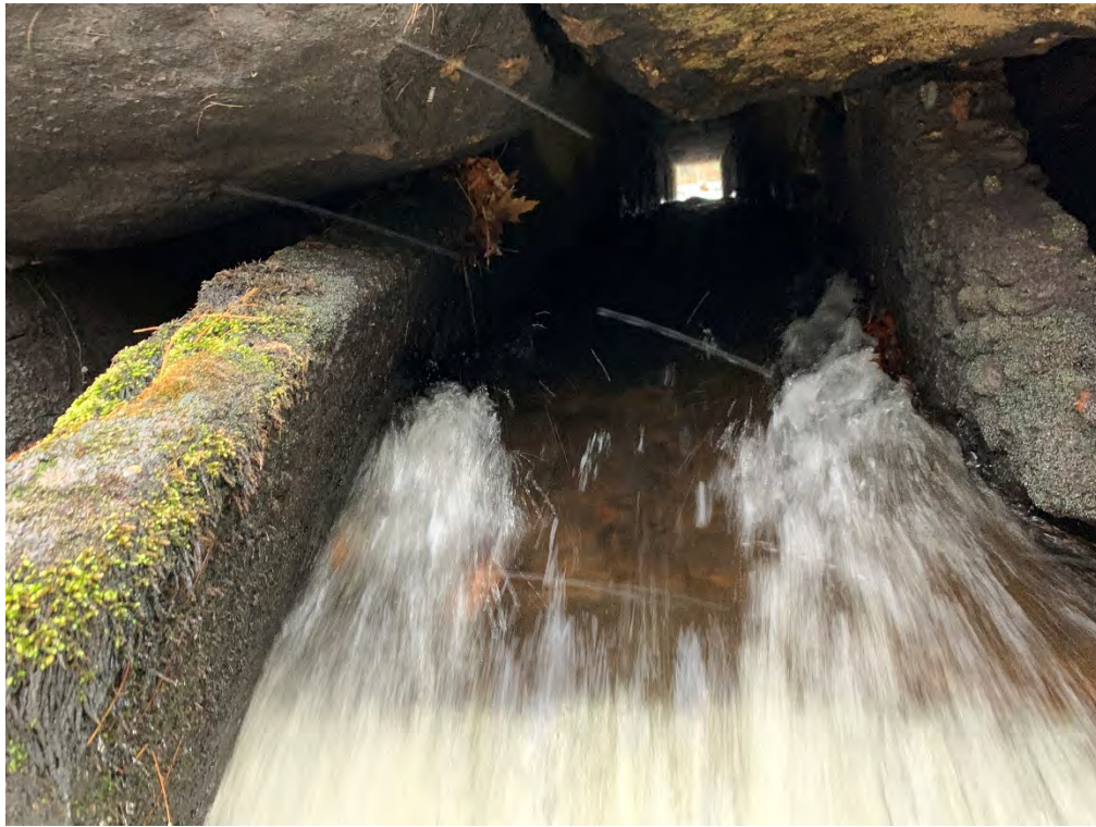
Photo 25 - The LLO conduit viewed looking upstream from the downstream end where the conduit daylights through the cascading boulder-lined slope. The conduit appeared to be flowing freely.
