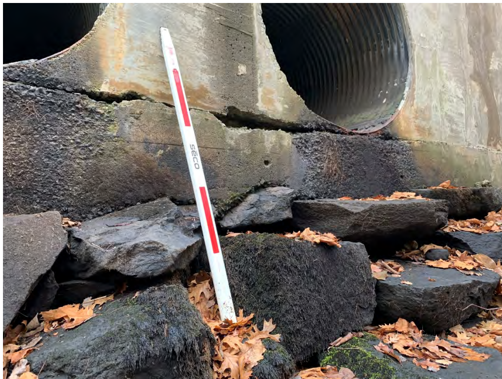
Photo 22 - Close-up view of cracked and deteriorated concrete at the spillway endwall along an apparent construction joint.
