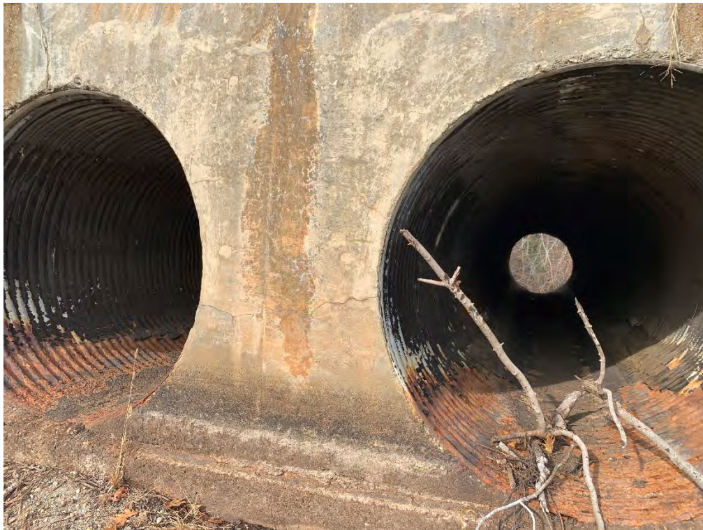
Photo 20 - Close up view of two of the CMPs. The protective bituminous coating on the CMPs is cracked at the top of the pipes and is missing along the inverts. The bottom of the CMPs are corroded where the bituminous coating is missing.
