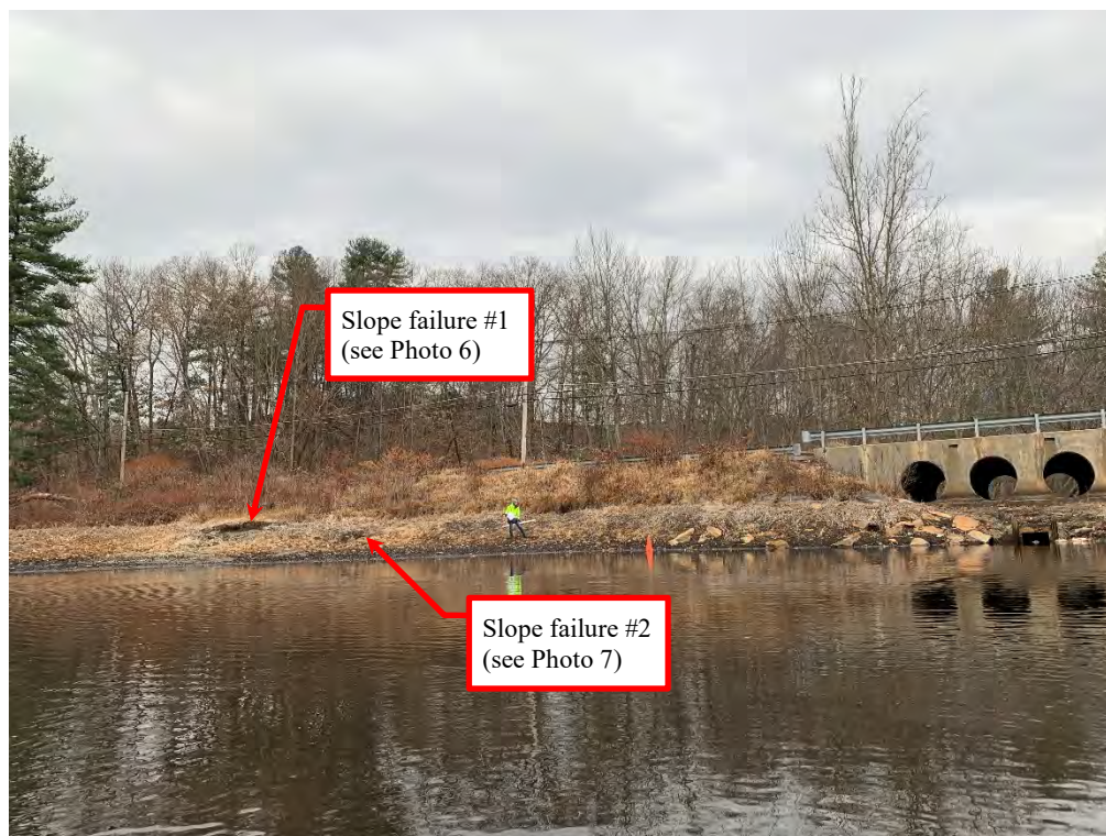
Photo 4 - Overview of the upstream slope (left of the spillway). Two isolated slope failures were observed below the normal pool elevation. Vegetation conditions were similar to those described in Photo 3.
