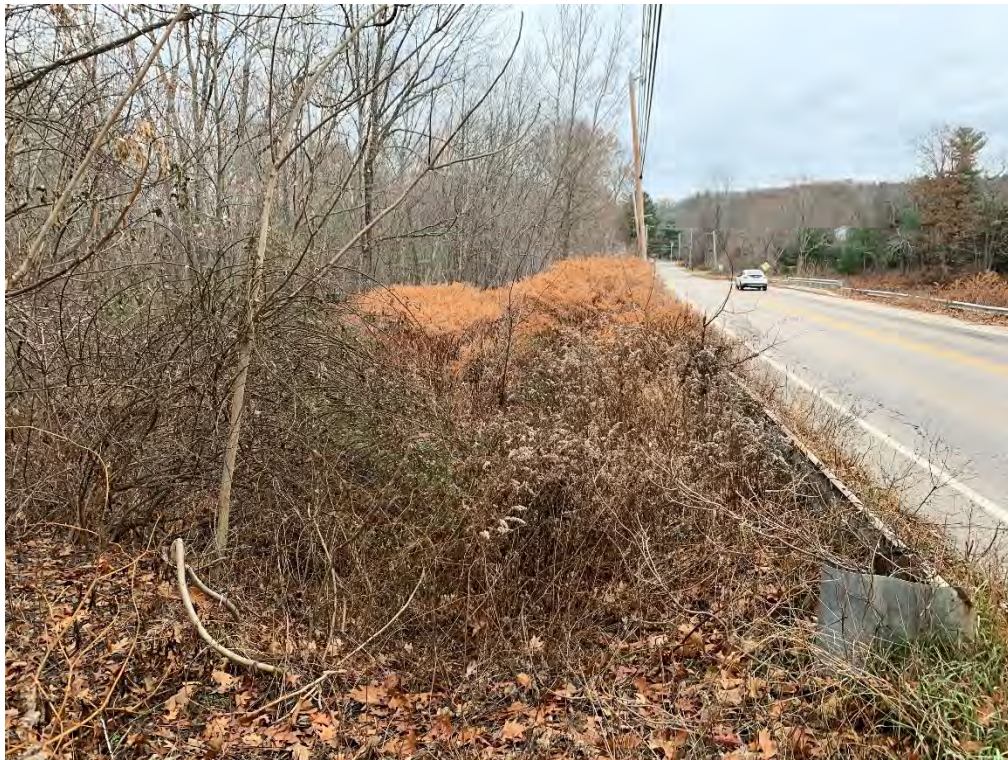
Photo 14 - The downstream slope where it contacts the left abutment (left downstream groin). Thick brush and wetland vegetation is present in this area.
