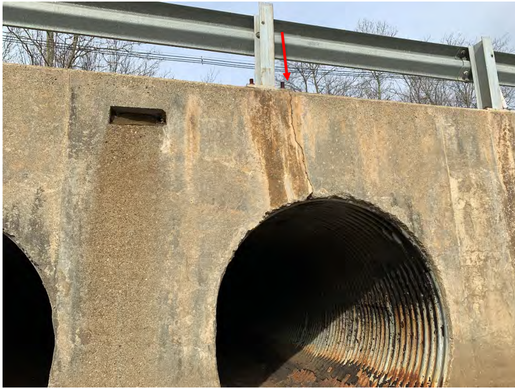
Photo 19 - Close up view of a transverse crack above rightmost CMP.
