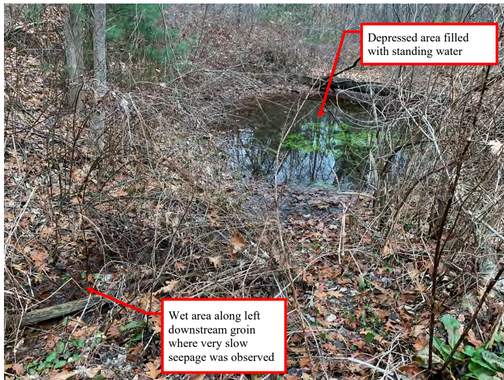
Photo 17 - Ponded water in a depression along the toe of the downstream slope near the left abutment. A wet area with slow seepage was observed upstream of the ponded water along the lower portion of the left downstream groin. Seepage has been observed in this area previously, but the origin/source is unknown.
