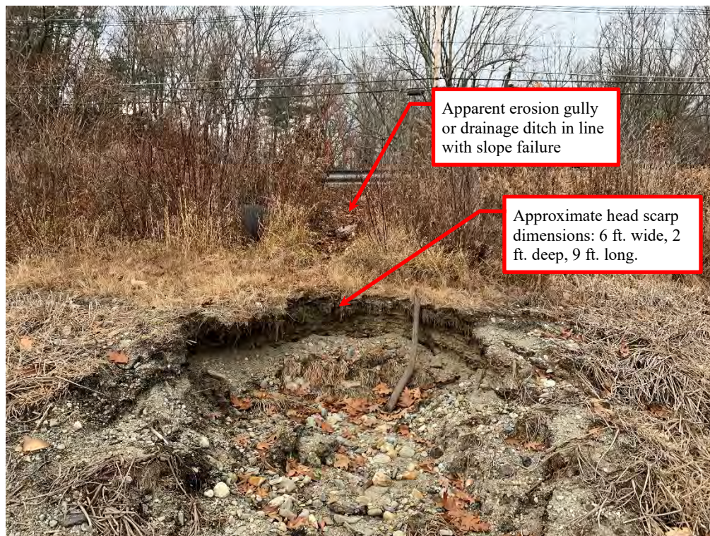
Photo 6 - Close-up view of slope failure #1 shown in Photo 4. An apparent erosion gully or drainage ditch is located above and in-line with the scarp.
