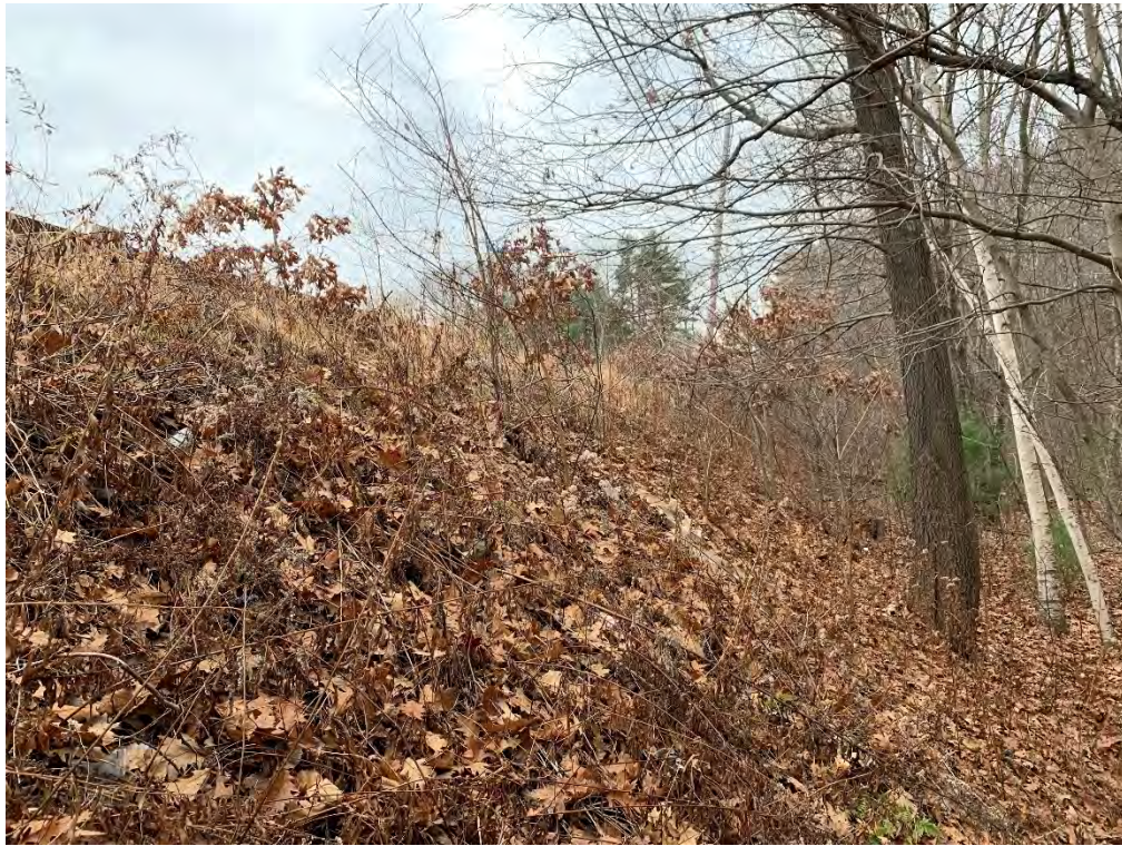
Photo 13 - The downstream slope between the spillway and right abutment. Woody vegetation and a thick cover of leaves and plant debris made inspection difficult and may have obscured deficiencies.
