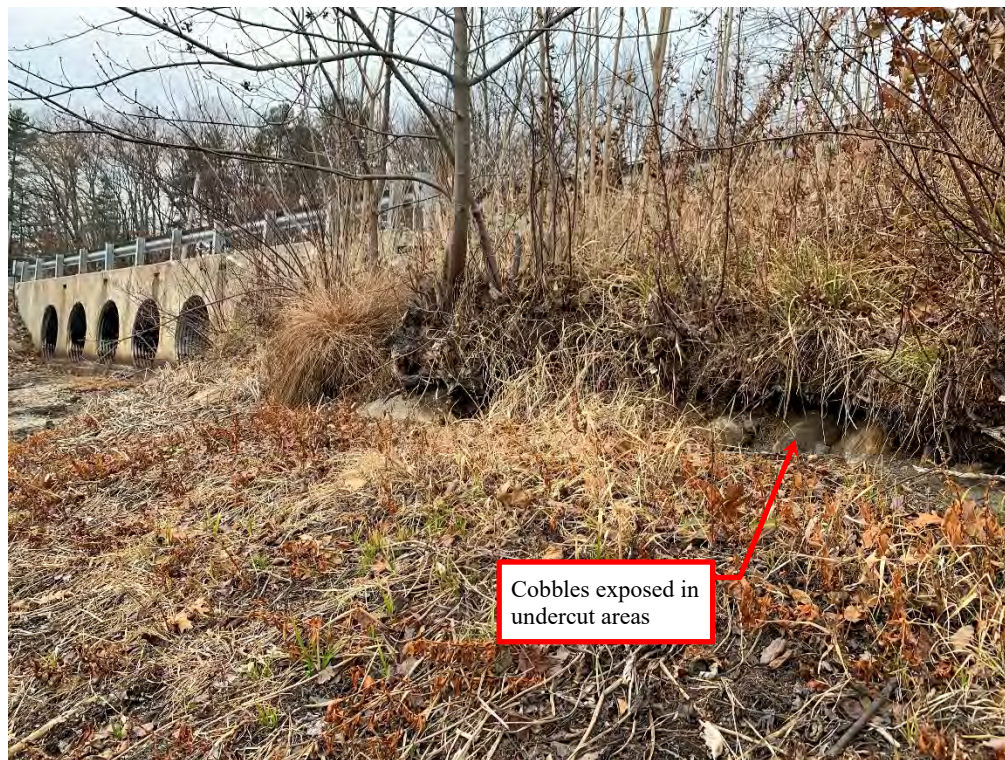
Photo 5 - The upstream slope near the spillway. As noted in Photos 3 and 4, an erosional scarp is present on the upstream slope along the normal pool elevation. The maximum height of the scarp was approximately 8 inches. Up to 12 inches of slope undercutting along the scarp was observed in several areas.
