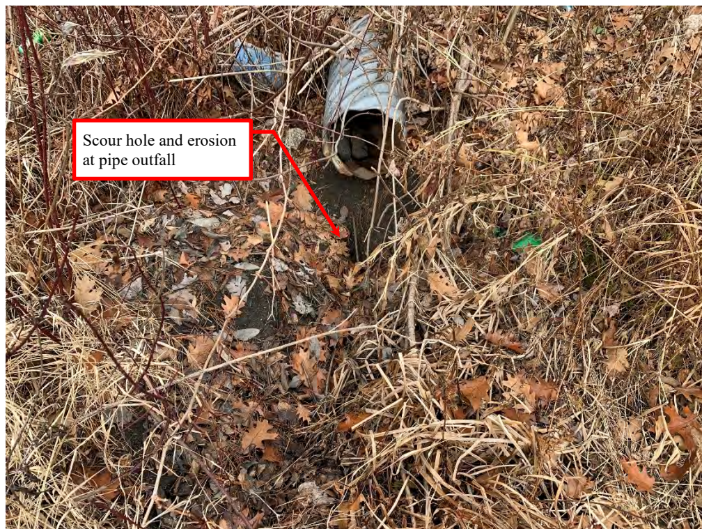
Photo 8 - The outfall of a 12-inch corrugated metal stormwater drain pipe connected to a catch basin on the dam crest. This outfall is located on the upstream slope between the spillway and left abutment.
