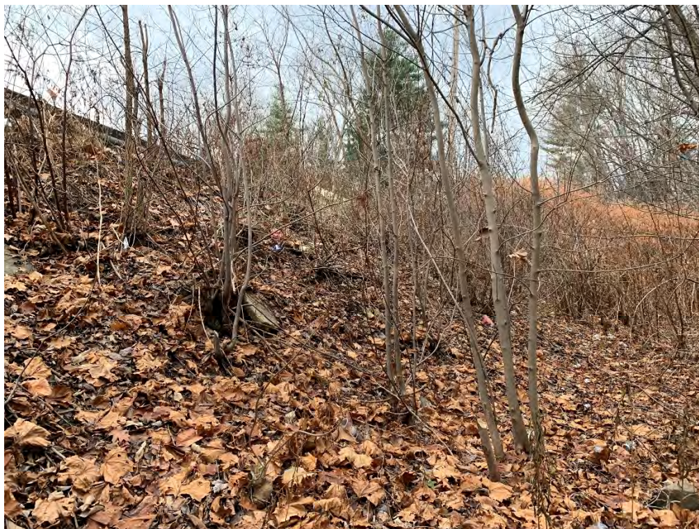
Photo 15 - The downstream slope between the spillway and left abutment. Woody vegetation and a thick cover of leaves and plant debris made inspection difficult and may have obscured deficiencies.
