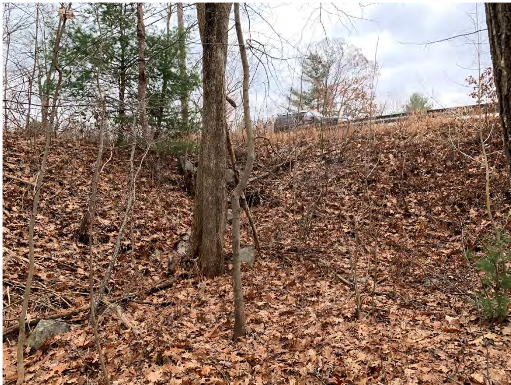
Photo 12 - The right end of the downstream slope where it contacts the right abutment (right downstream groin). Woody vegetation and large trees are present.
