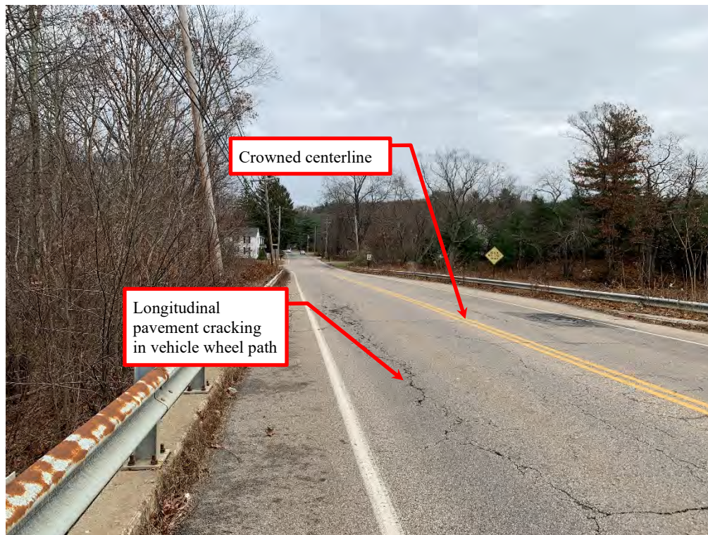
Photo 9 - Overview of the dam crest (Boston Road) from the spillway, facing the right abutment.
