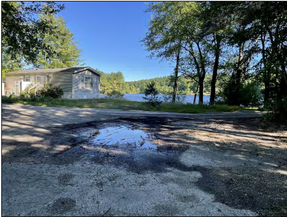
Photo No. 3.: Upper Tucker Pond South Dam low area at right end of dam that serves as informal auxiliary spillway (a.2)
