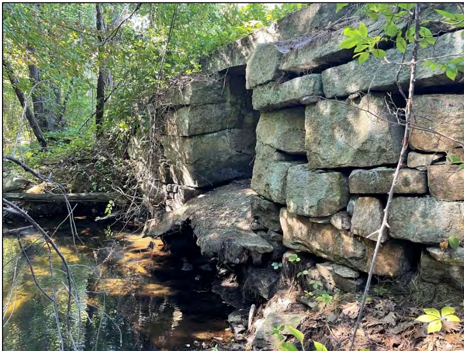
Photo No. 2.: Upper Tucker Pond East Dam discharge end of spillway culvert (a.1)
