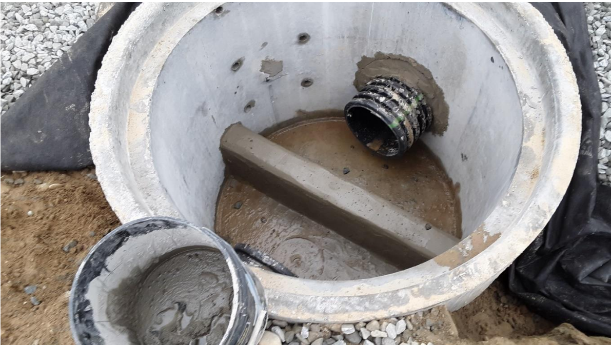
Photo 2: A weir wall had been built within the outlet control structure.
