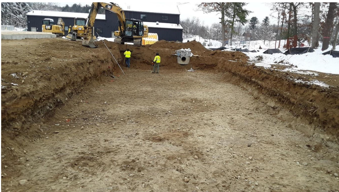
Photo 1: The bottom of the excavated area for the subsurface infiltration system had been scarified in a satisfactory manner.
