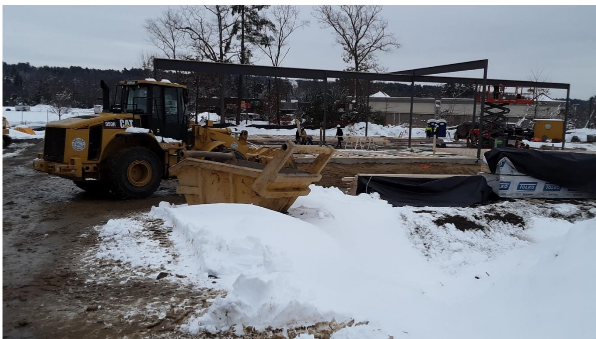
Photo 2: The contractor was installing the frame of the building.
