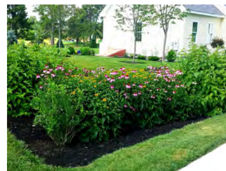
This rain garden in Devens, MA gathers runoff from a curb-less road and sidewalk to infiltrate stormwater back into the ground while also offering beautiful home landscaping. Rain gardens can be made in any size and shape to fit your location.
