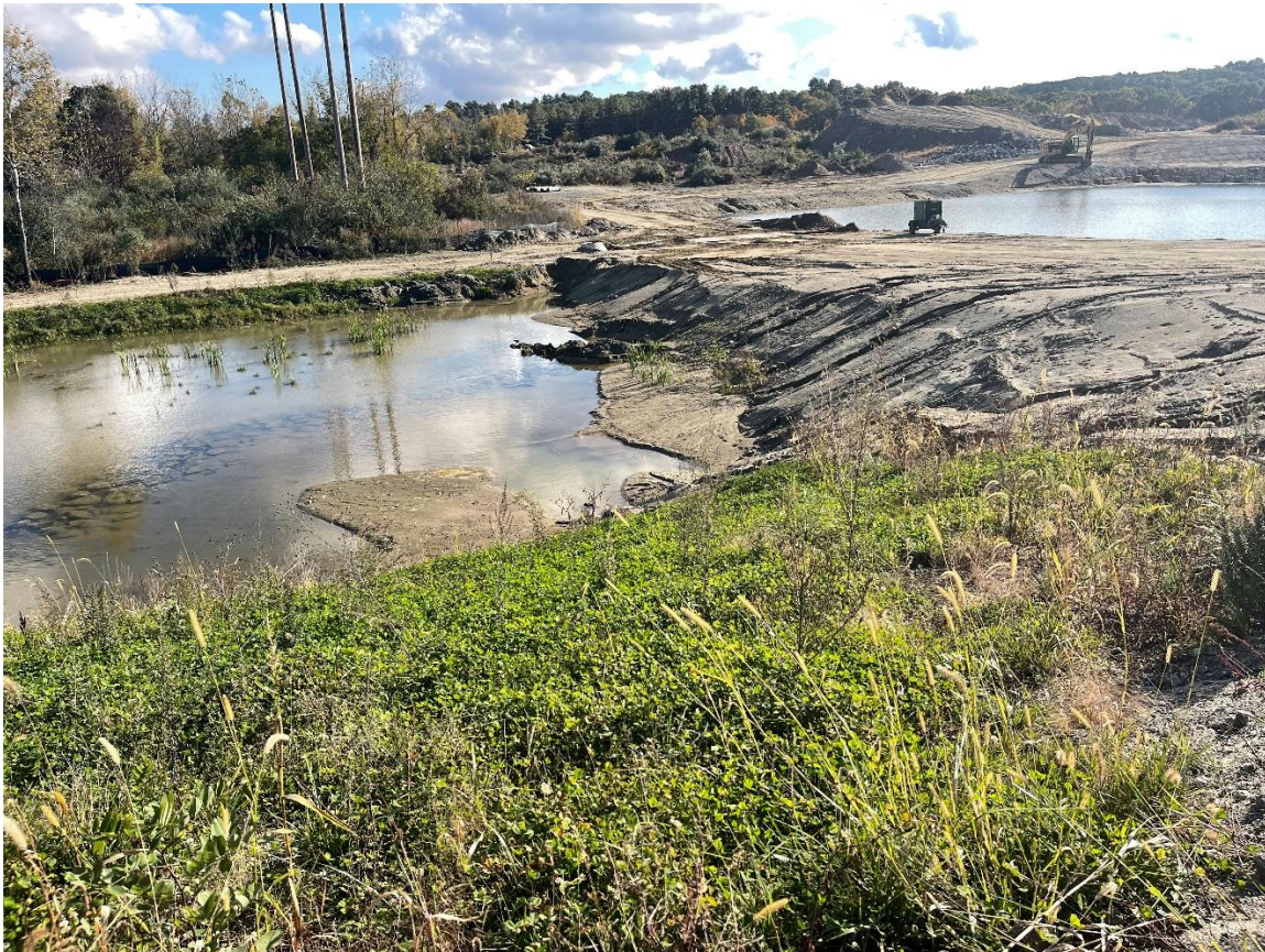
Photo 1: The erosion rills at the southern corner of SWMA #3 have not been repaired yet, nor the sediment cleaned.
