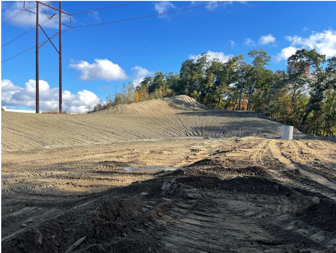
Photo 2: Additional erosion rills have formed along the northern and eastern slopes of SWMA #4.
