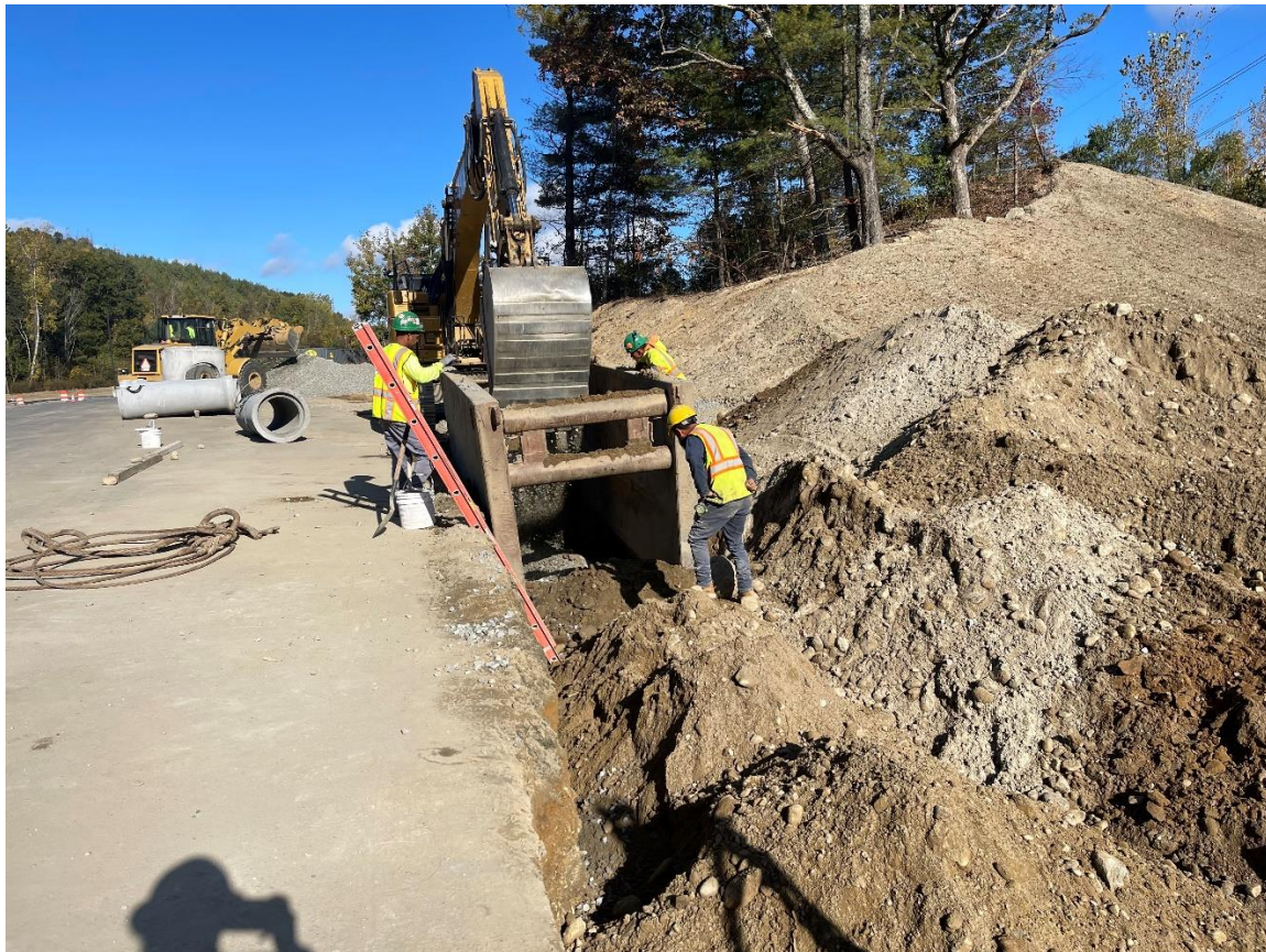
Photo 3: The contractor placing three-quarter-inch crushed stone over the pipe between DMHs 11 and 10.
