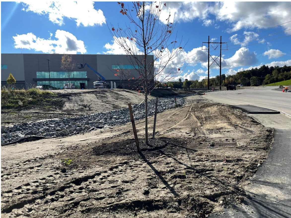
Photo 6: Additional riprap had been placed along the swale on the western side of Lot 3.
