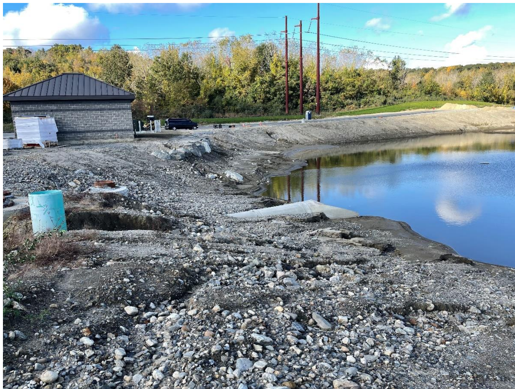
Photo 2: The erosion rills on the southern side of SWMA B3a have worsened.
