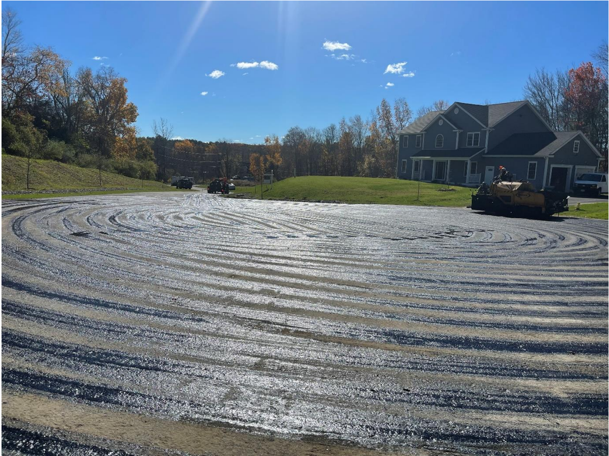
Photo 1: Tack-coat placed on the cul-de-sac.
