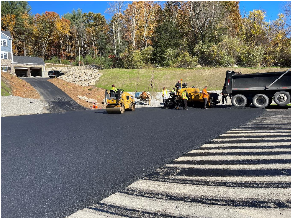
Photo 2: The contractor paving the right side of the cul-de-sac at approximately station 4+00. The contractor can also be seen compacting the asphalt with a 3-5-ton roller.
