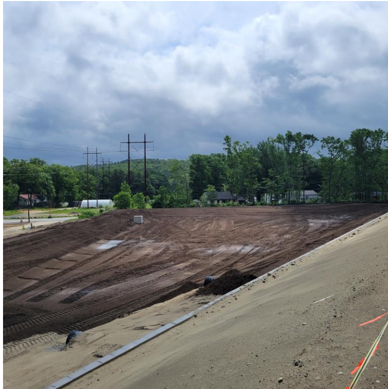
Photo 3: Infiltration Basin 1 with loam spread.
