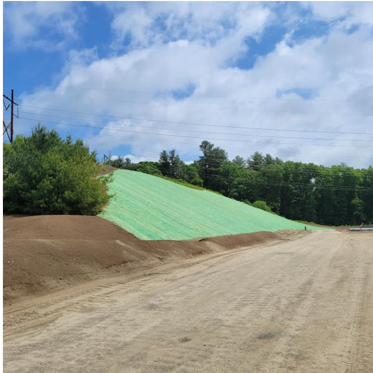
Photo 2: Erosion control matting installed along the northern 2:1 slope.
