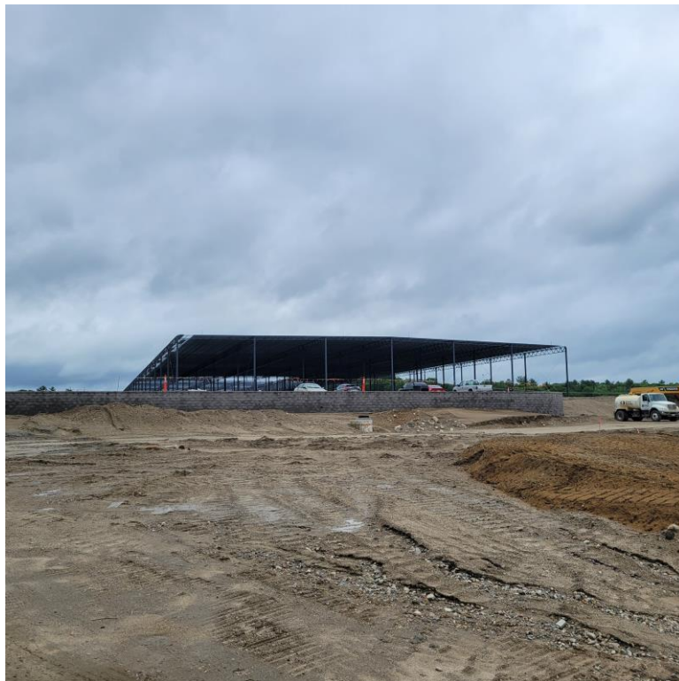
Photo 4: General condition of building construction with southern retaining wall installed.
