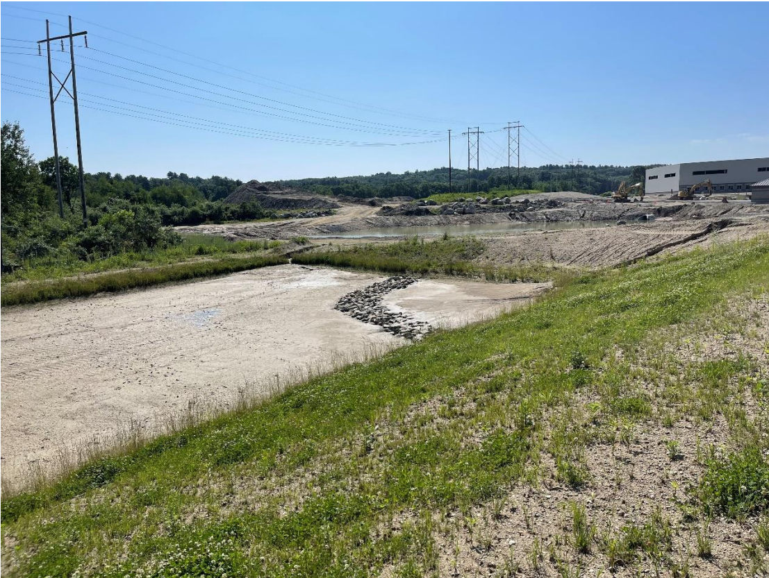
Photos 1 and 2: SWMA #3 was experiencing partial grass growth along its slopes and no grass growth along the southwestern corner and bottom.
