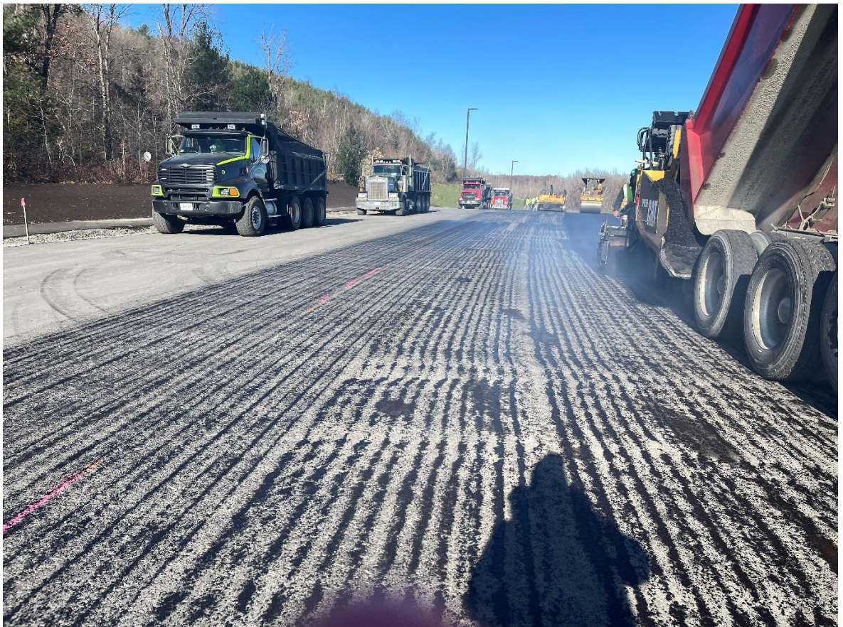
Photo 2: Tack coat was placed along the roadway.
