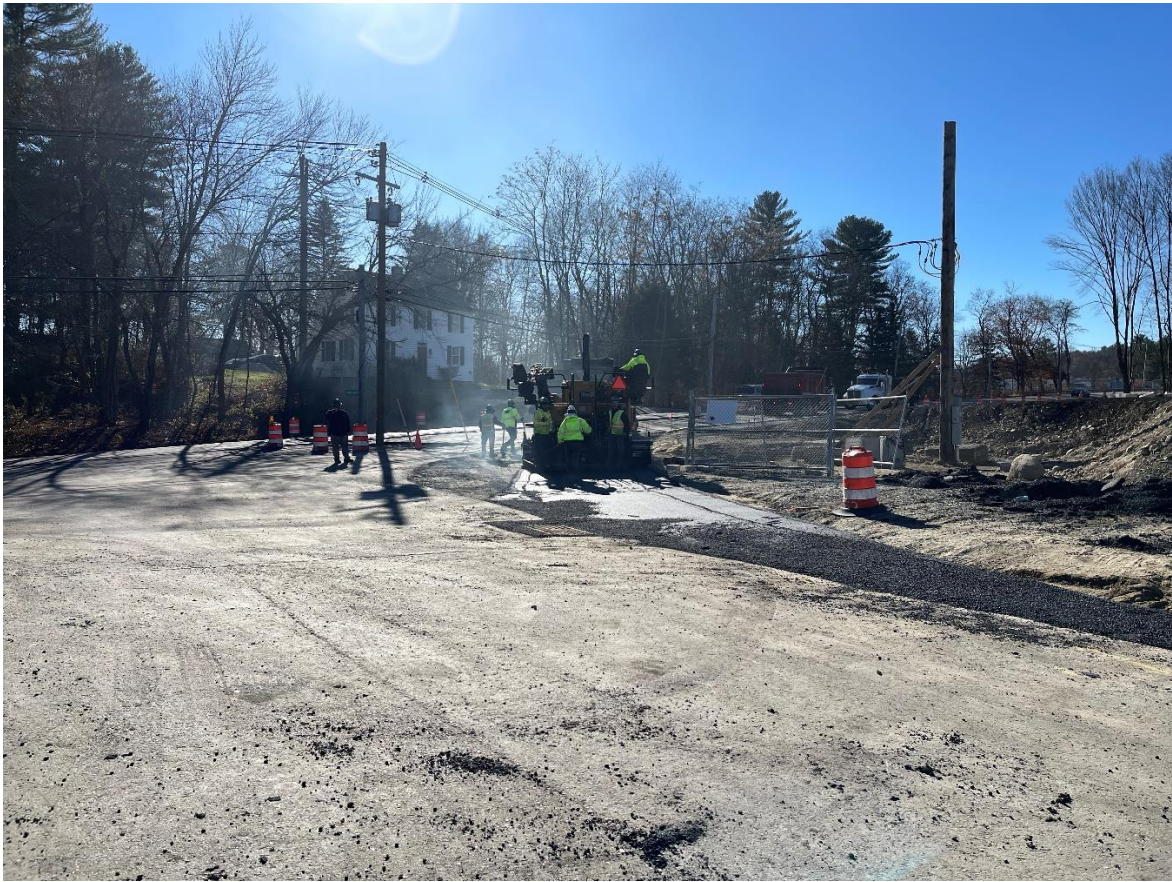
Photo 3: The contractor paving the temporary turning lane at Boston Road.
