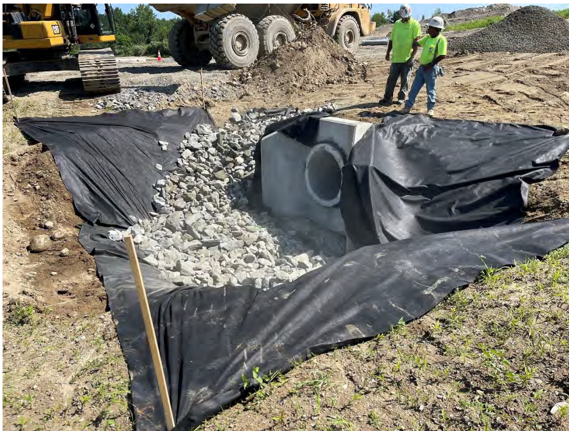
Photo 3: The contractor placing riprap around HW 600.
