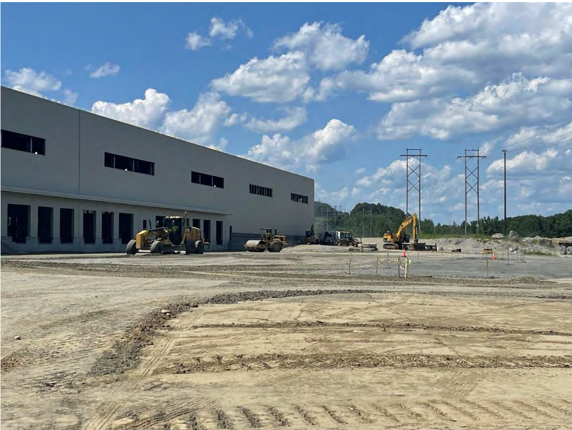
Photo 2: The contractor fine-grading and compacting the eastern parking lot.
