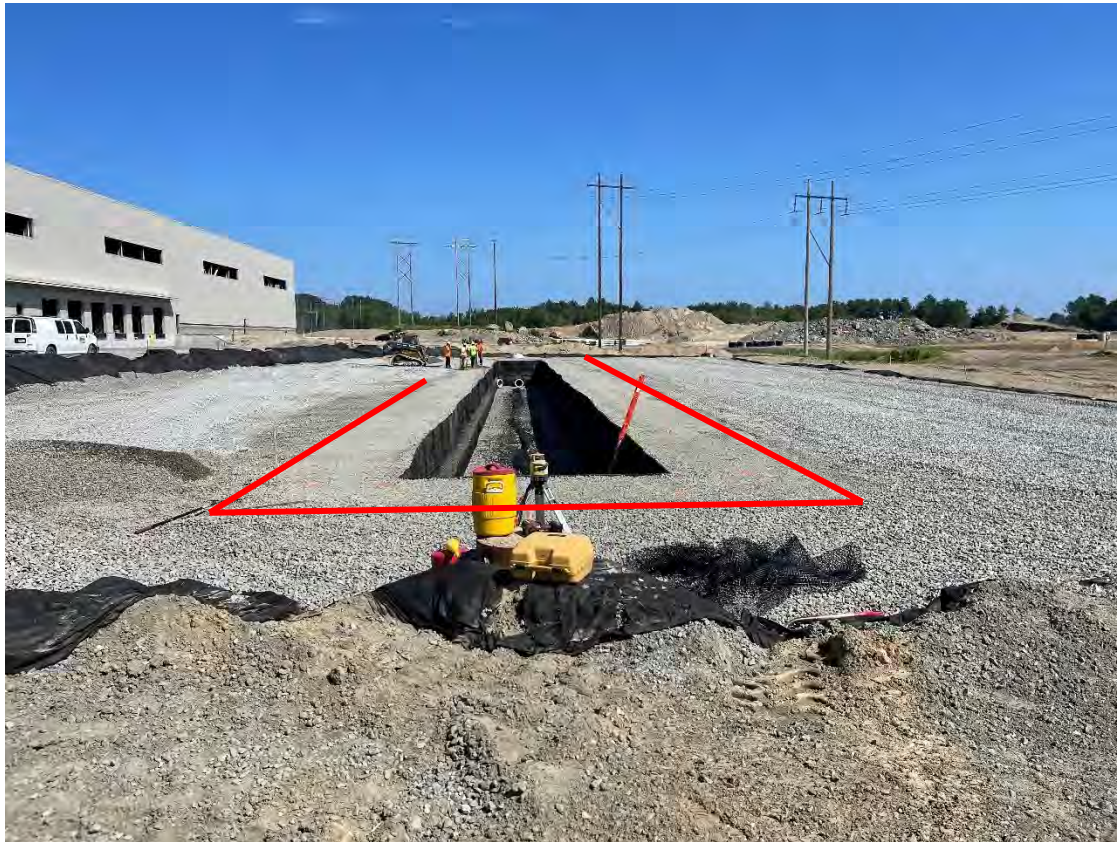
Photo 2: Overall progress of SWMA UG3c. A red line has been added to show the separation between the three-quarter-inch and one-and-a-half-inch crushed stone.
