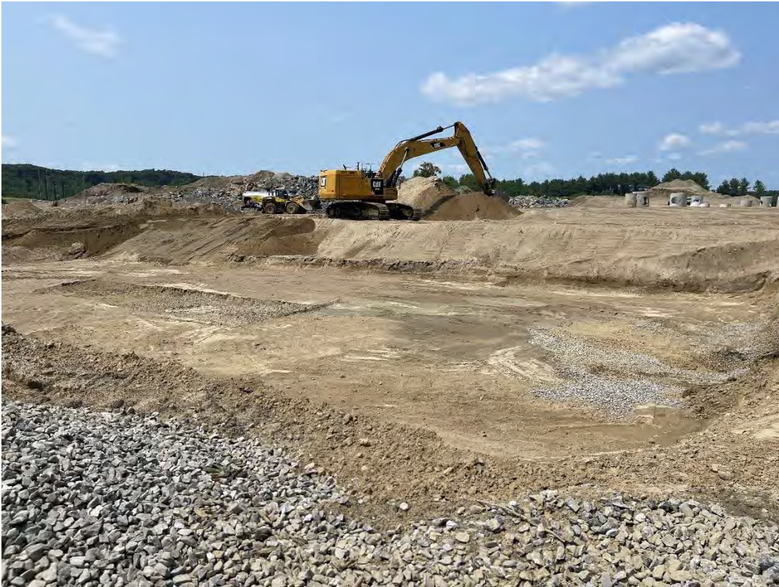
Photo 3: The contractor placing fill material along the northern slope of SWMA UG2e.
