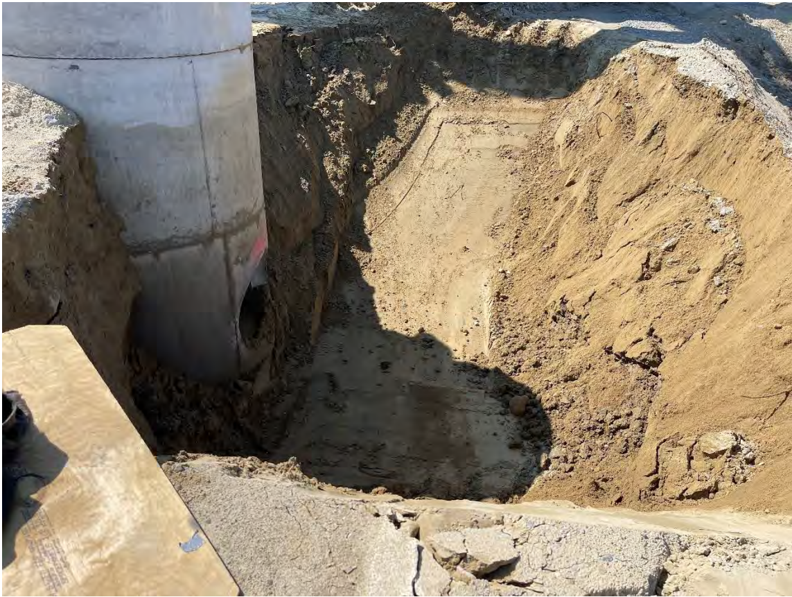
Photo 4: The contractor was excavating the trench for the pipe between OCS 500 and SWMA UG2e.
