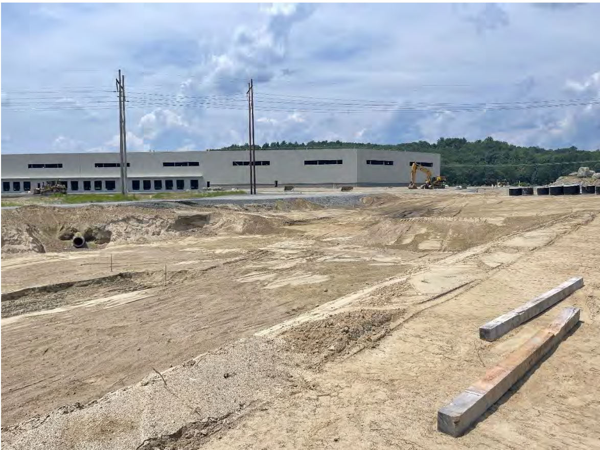
Photo 3: SWMA UG2e was further excavated. The width increased to 160 feet where the pipe from DMH 503 intersects with the stormwater management area (middle left).
