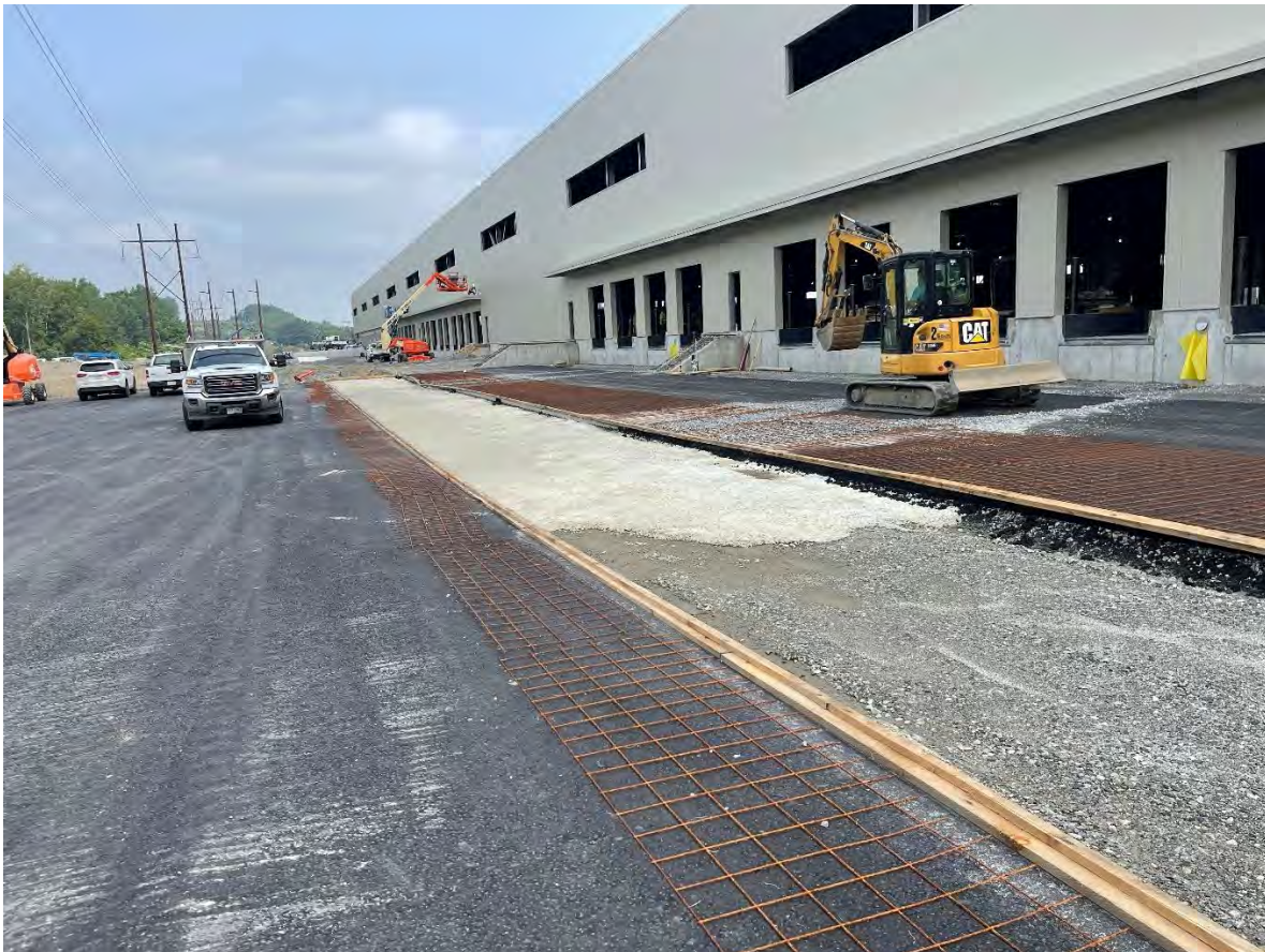
Photo 1: Approximately half of the concrete for the pad adjacent to the southern portion of the western side of the building had been poured.
