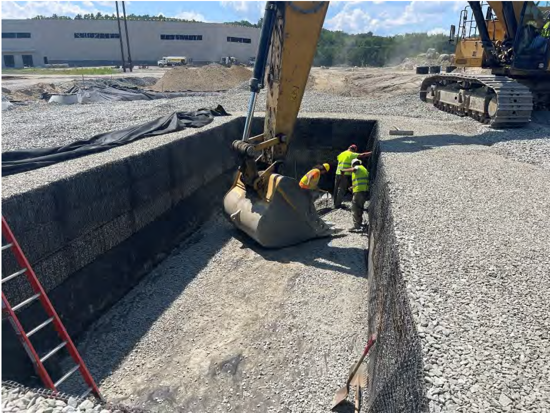
Photo 3: The contractor removing excess crushed stone that had fallen into the trench of SWMA UG2e. Geogrid is visible along the sides of the trench, and the top of the reinforced zone can be seen adjacent to the trench.
