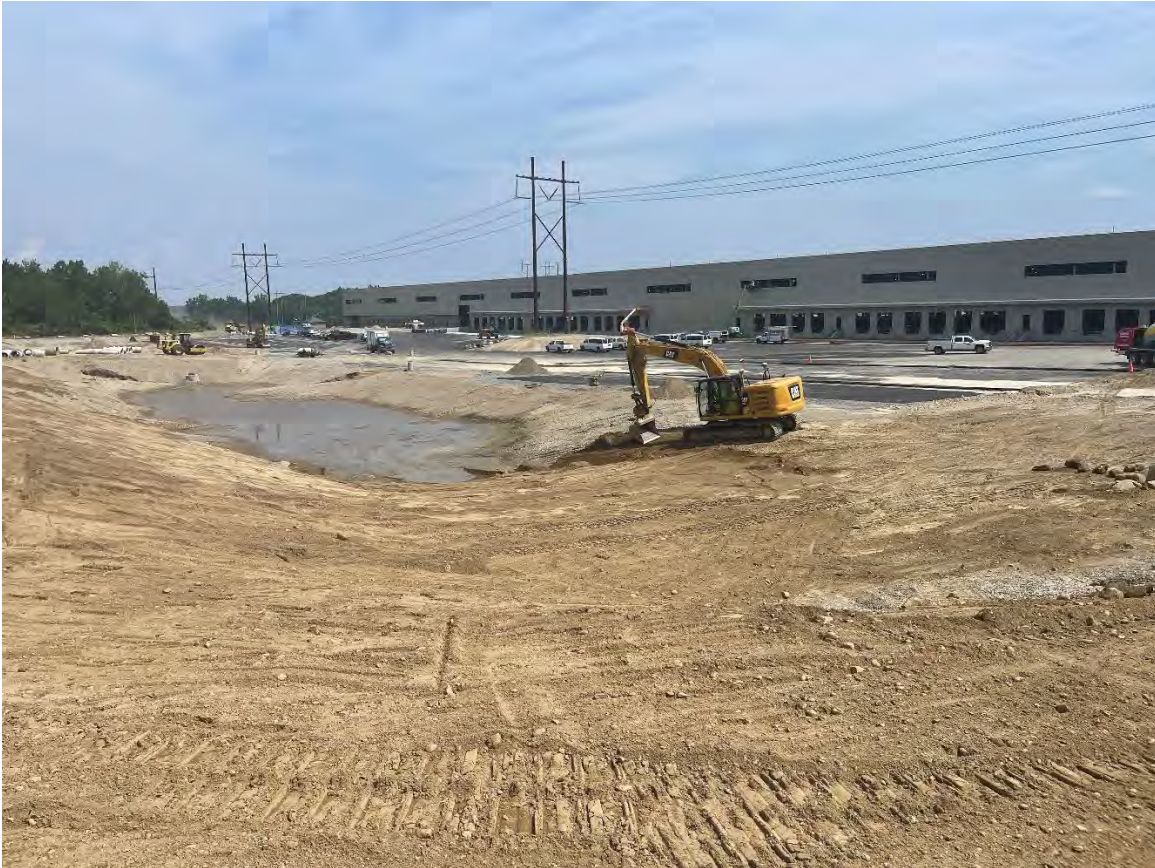
Photo 1: The contractor placing fill material along the slopes of BA 3b.
