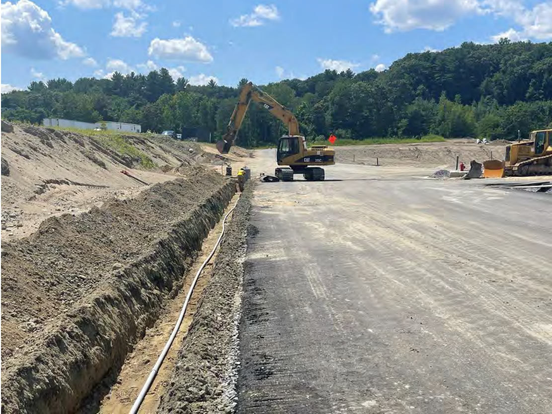
Photo 1: The contractor backfilling electrical conduit pipe along the road eastmost of Building 3.
