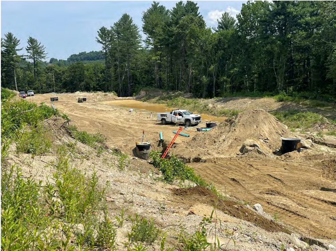
Photo 2: SMHs 106 and 107 were installed, and the pipe between them backfilled.
