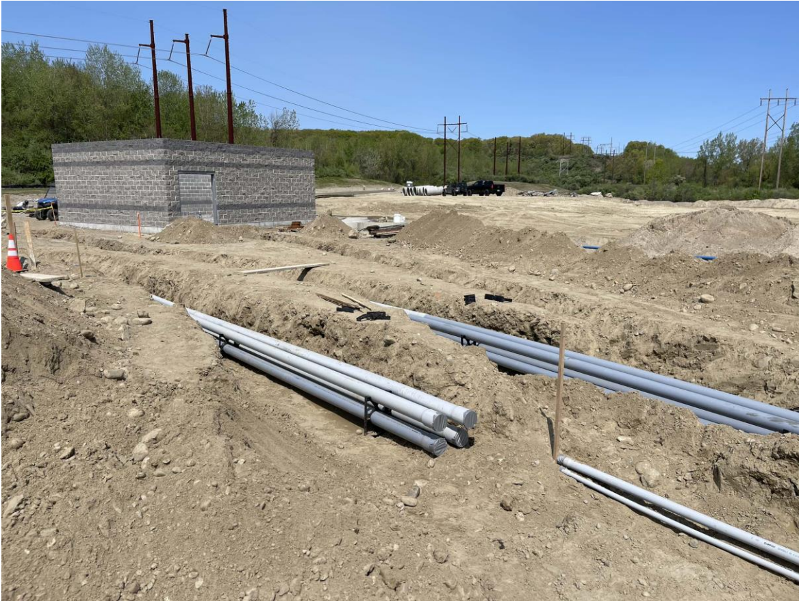
Photo 1: Electric conduit had been installed from the pump house towards Building 3.
