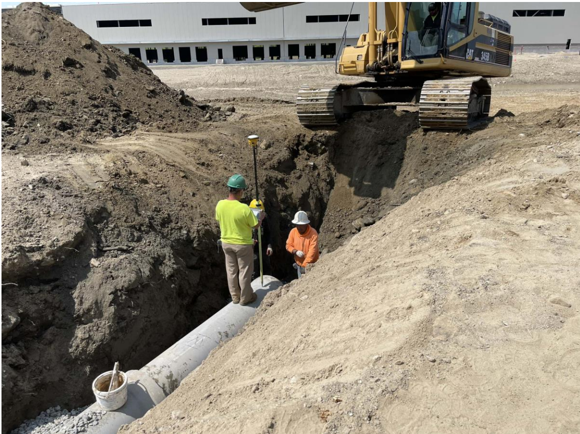
Photo 2: The contractor confirming the elevation of the pipe between DMH 807 and DMH 807A.
