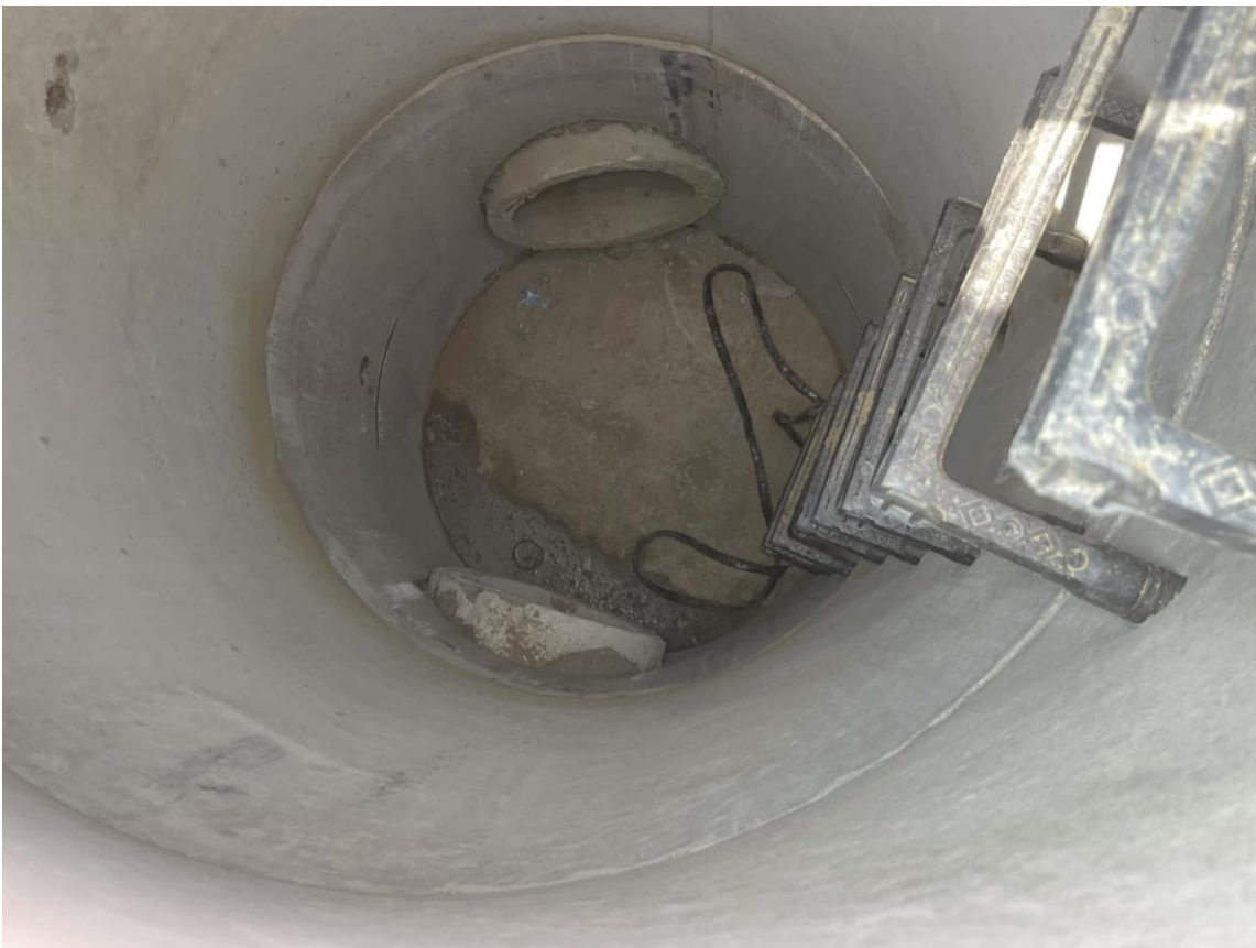
Photo 2: The pipe connection in DMH 807A for the pipe leading towards DMH 807 (bottom pipe in photo) was sealed with mortar.
