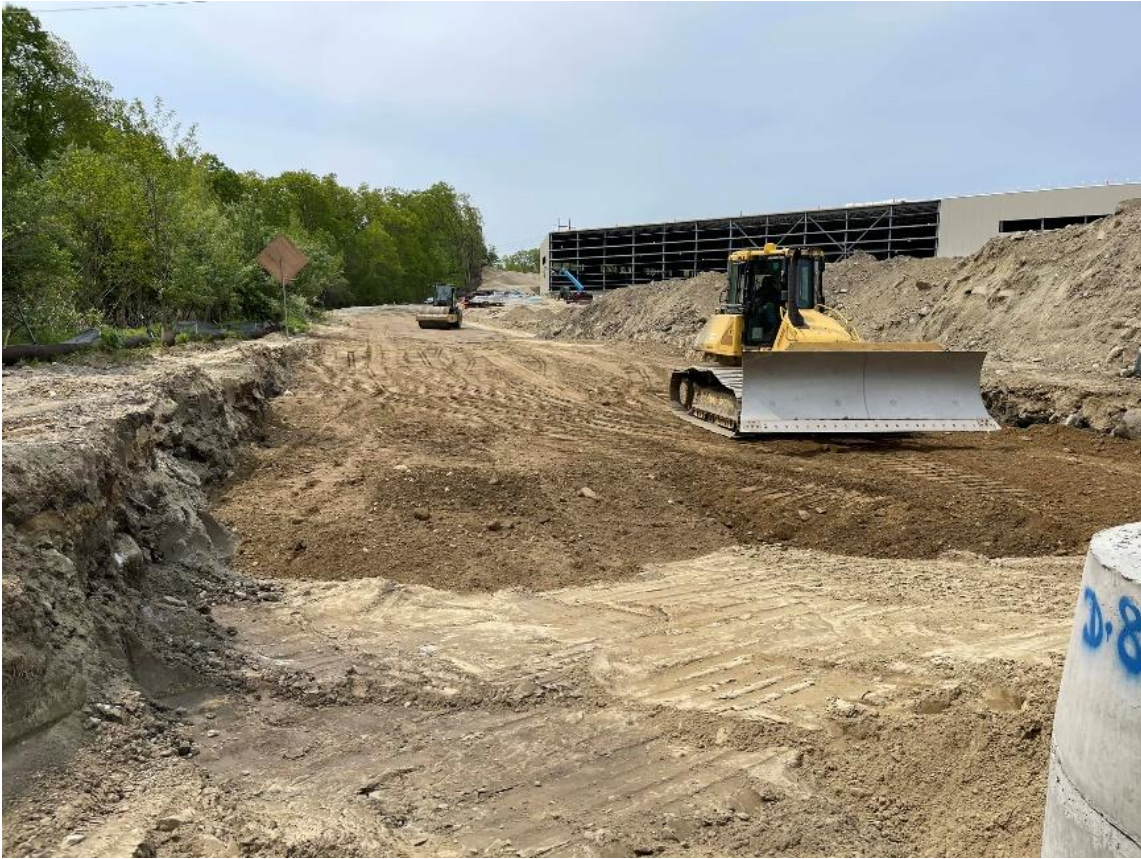
Photo 1: The contractor was placing fill material along the roadway adjacent to DMH 807.
