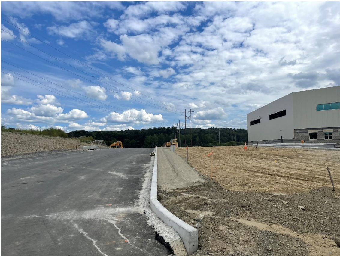
Photo 2: The area for the sidewalk along the northern driveway leading to the back roadway of the site had been prepared, and precast concrete curb installed. The contractor can be seen spreading fill material in the distance.
