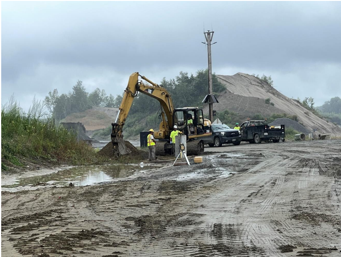
Photo 4: The contractor installing a light pole base at station 23+50.
