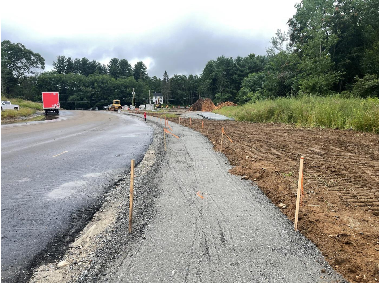
Photo 1: Dense grade crushed stone was placed and compacted along the sidewalk between stations 35+50 and 53+30.
