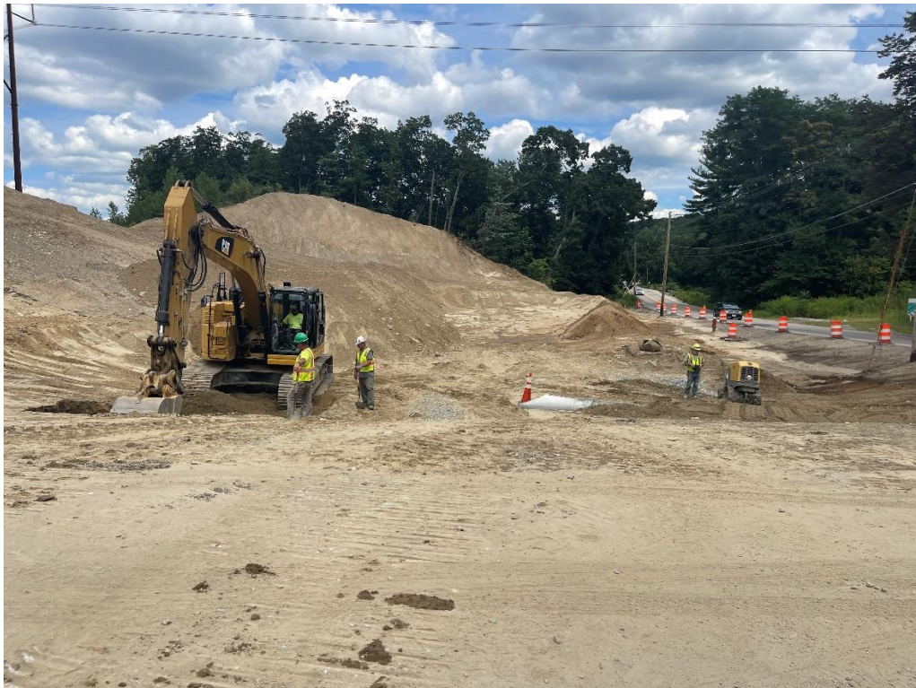
Photo 2: The contractor excavating SWMA #4 and backfilling the drainage pipe.
