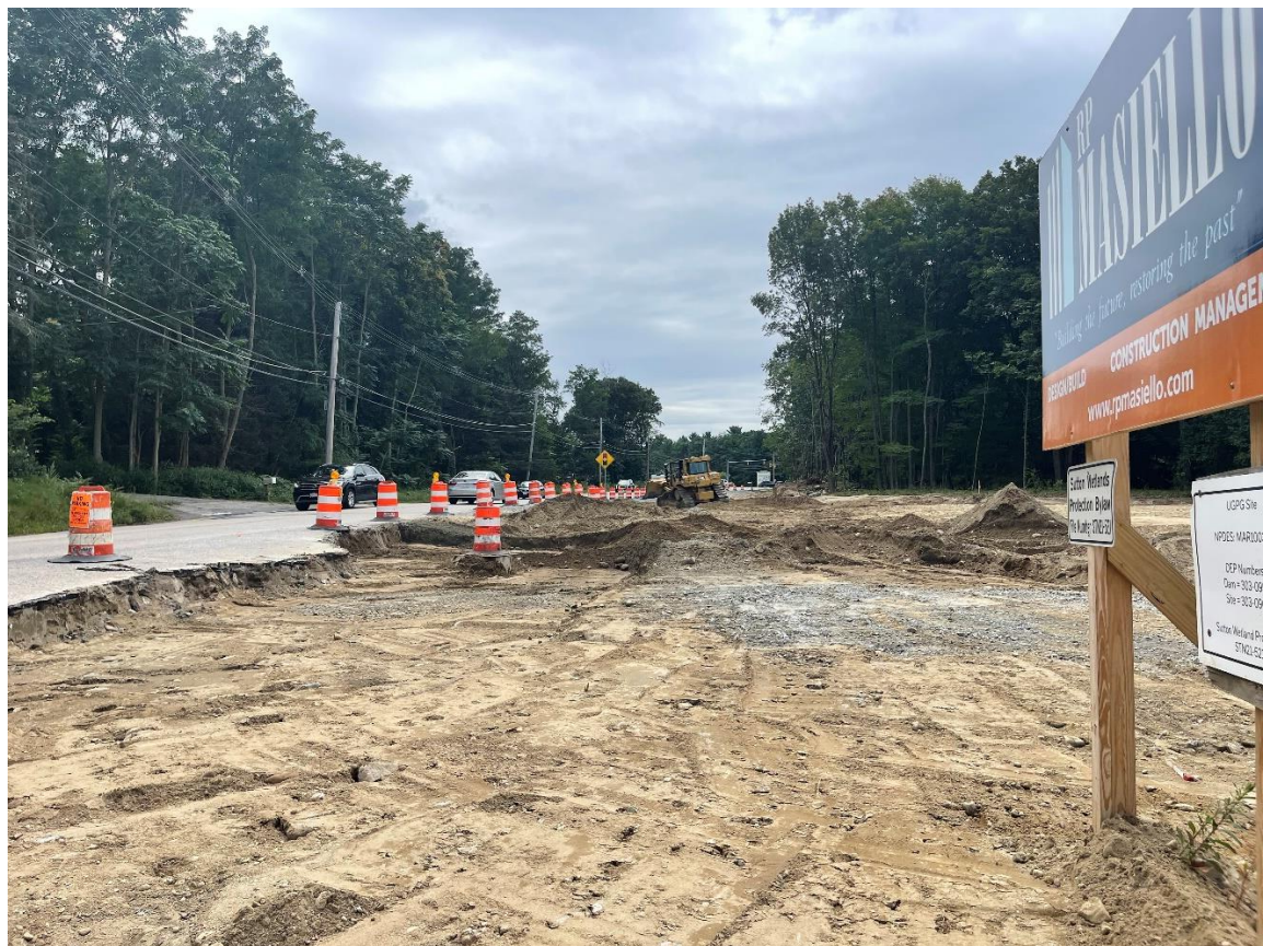
Photo 4: The contractor excavating and moving earth material in the Boston Road modification area west of the entrance.
