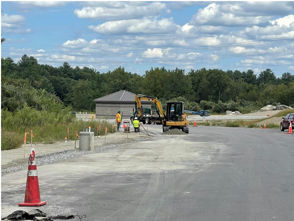
Photo 3: The contractor spreading dense grade crushed stone along the sidewalk.
