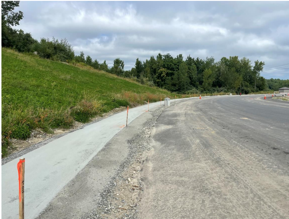
Photo 3: The sidewalk had been fine-graded.
