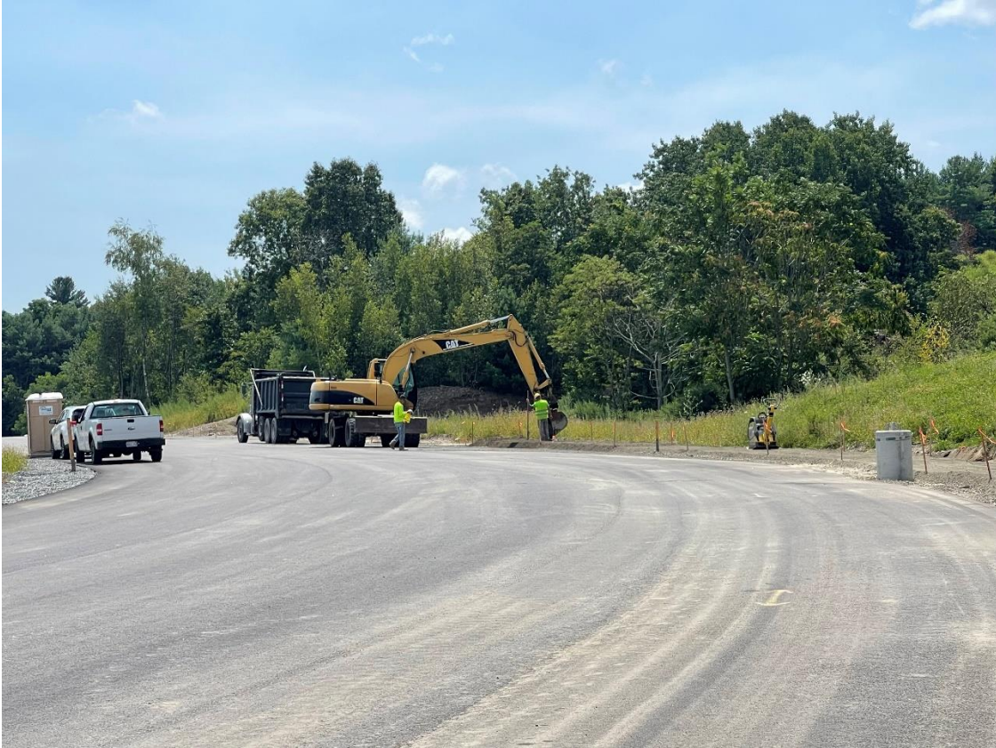
Photo 1: The contractor placing dense-graded crushed stone at station 46+00.
