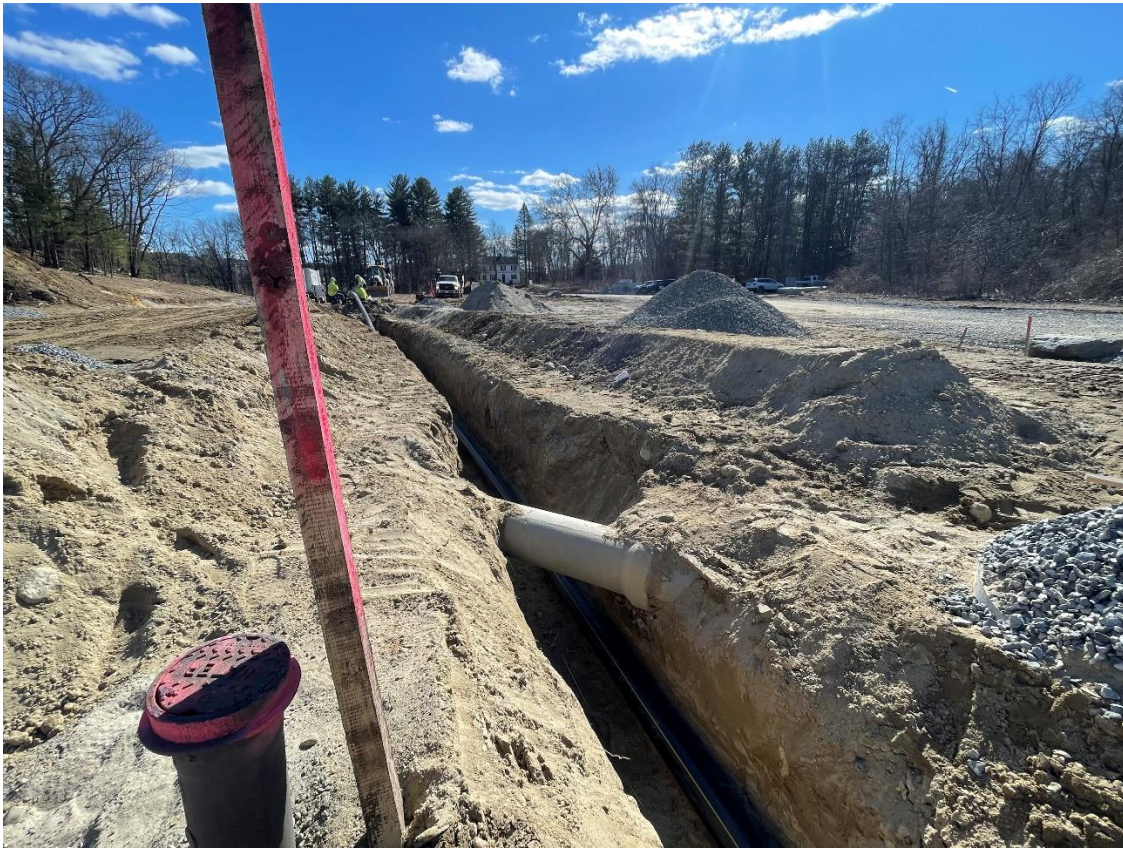
Photo 1: At approximately station 53+75, the contractor was installing gas utility pipe. There was approximately six inches of space between the drainage pipe and gas pipe.
