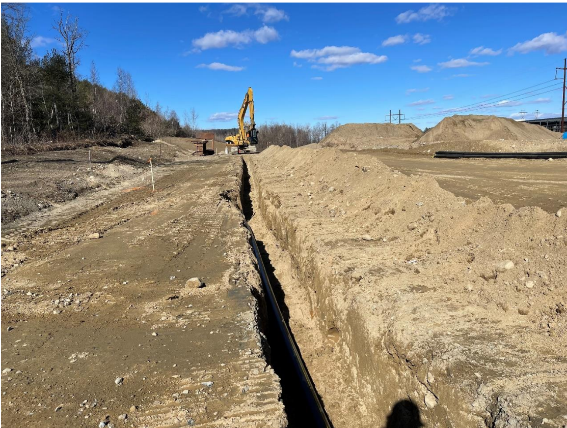
Photo 2: The gas utility pipe had been installed until station 51+00. At station 50+00, the contractor was excavating the utility trench.
