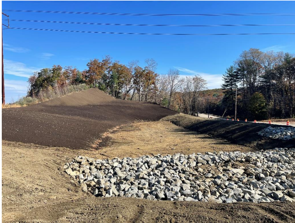
Photo 3: Loam had been placed along the northern and eastern slopes of SWMA #4, as well as the berm. The forebay and emergency spillway stones are also visible.
