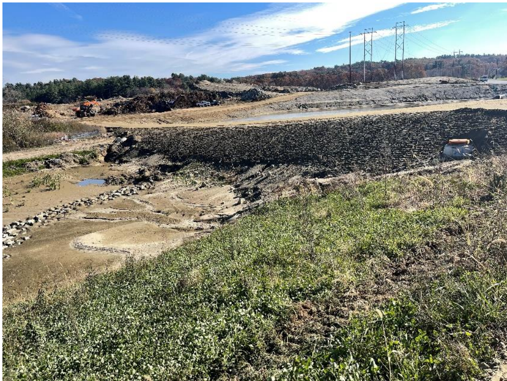
Photo 2: Loam had been placed along the southern slope of SWMA #3, and the erosion rills were repaired.
