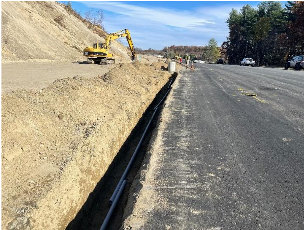
Photo 1: The contractor installing electrical conduit between stations 15+00 and 23+00.
