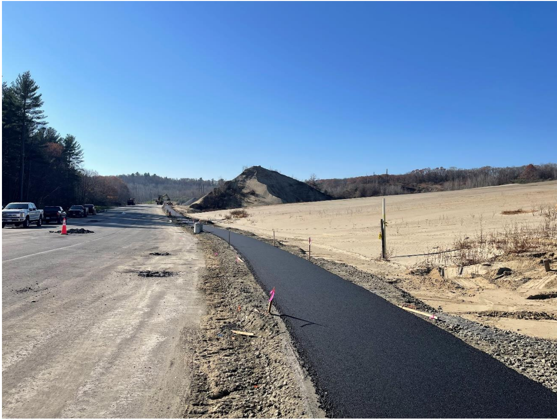
Photo 3: The binder course asphalt of the sidewalk between stations 1+00 and 13+00 had been paved and compacted.
