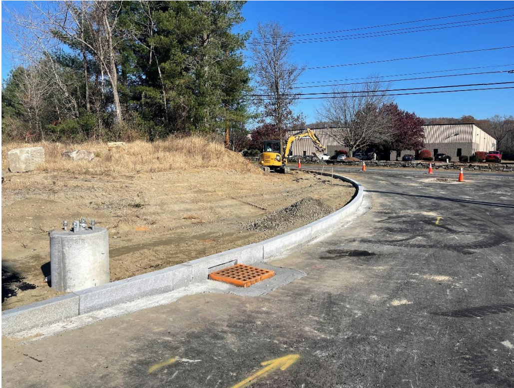
Photo 1: Vertical granite curbing had been installed at the Providence Road entrance.
