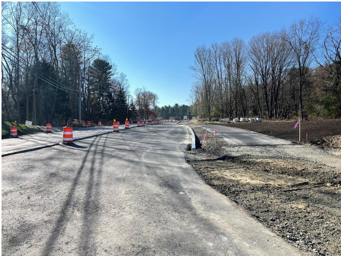
Photo 4: The binder course asphalt of the sidewalk along Boston Road had been paved, and vertical granite curbing installed. Barrels were placed on either side of the existing roadway.
