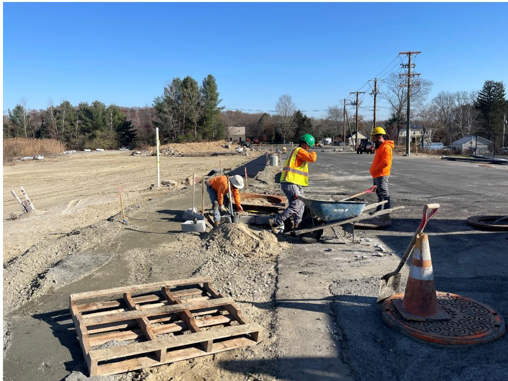
Photo 2: The contractor raising the casting of the electrical manhole at station 3+75.
