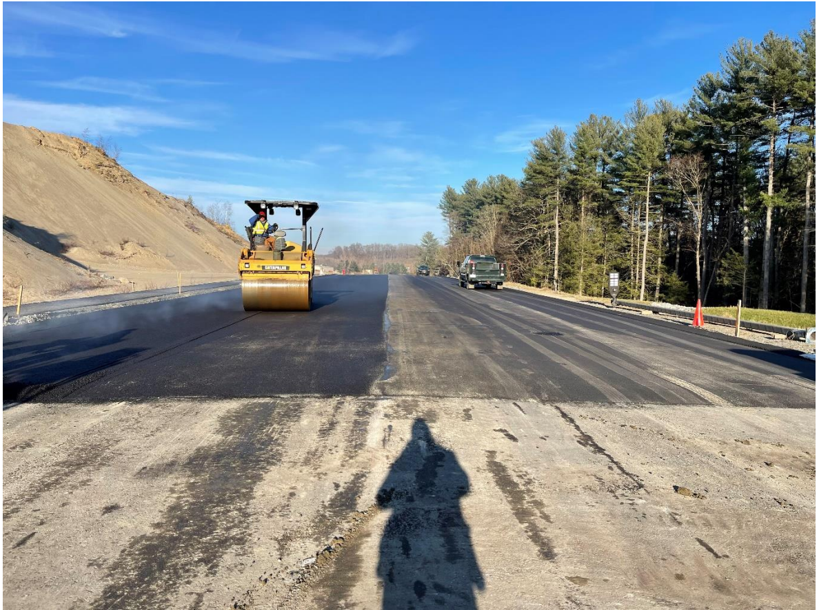
Photo 3: The contractor compacting the asphalt at station 16+40.
