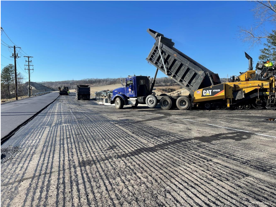
Photo 1: Tack coat was placed along the paved portion of the roadway.
