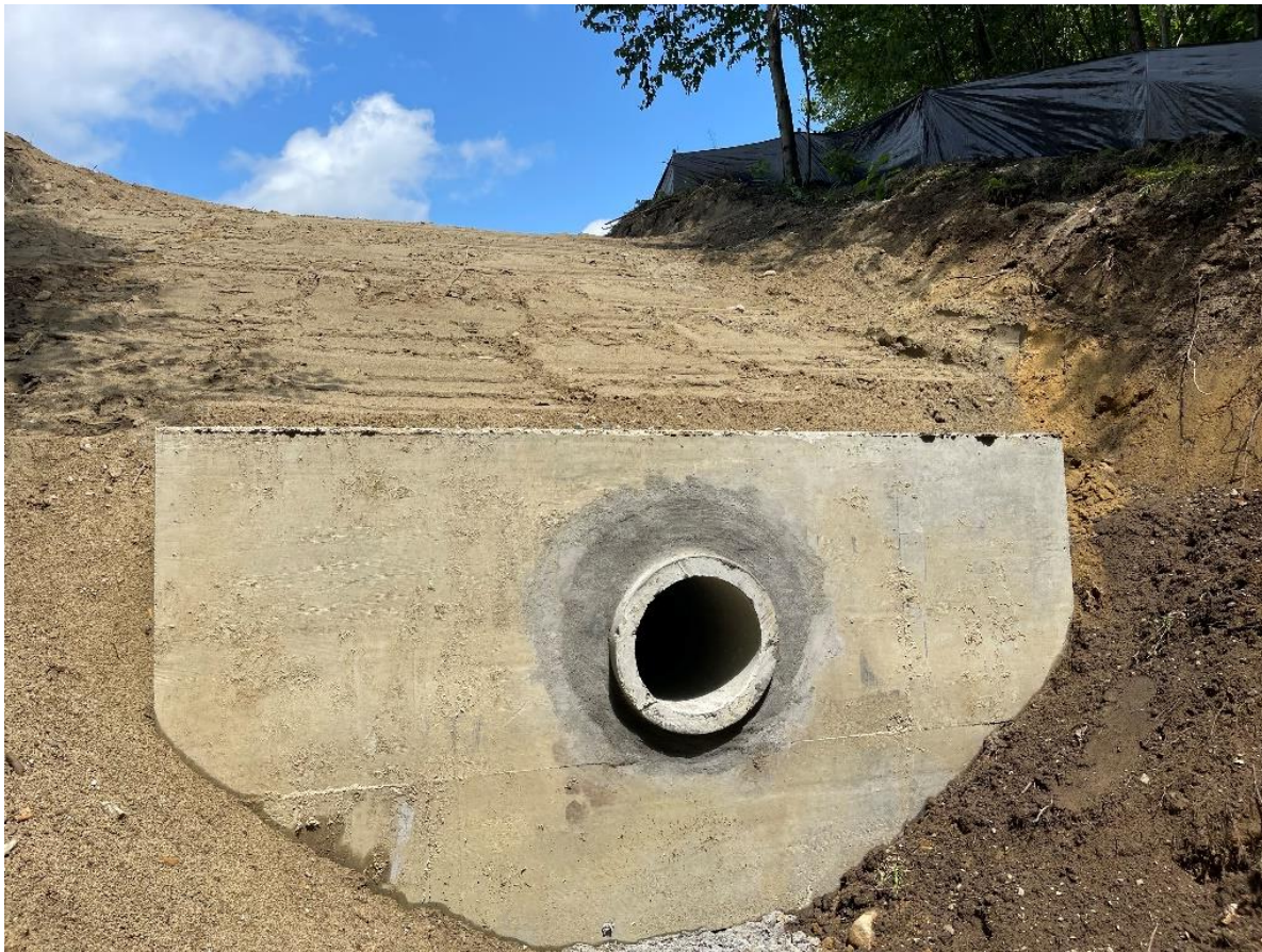
Photo 2: HW 500 was installed and its pipe connection sealed with mortar.
