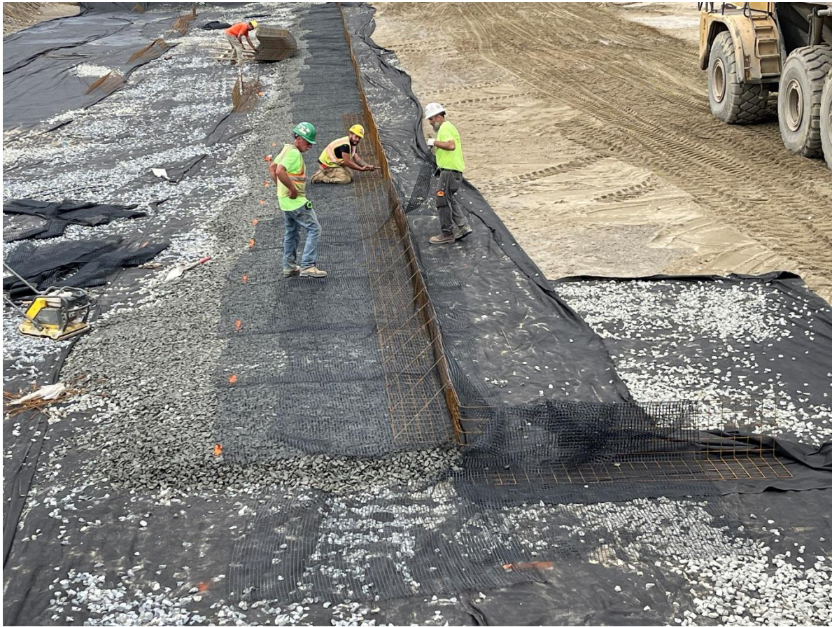
Photo 2: The contractor installing the second row of wire baskets.
