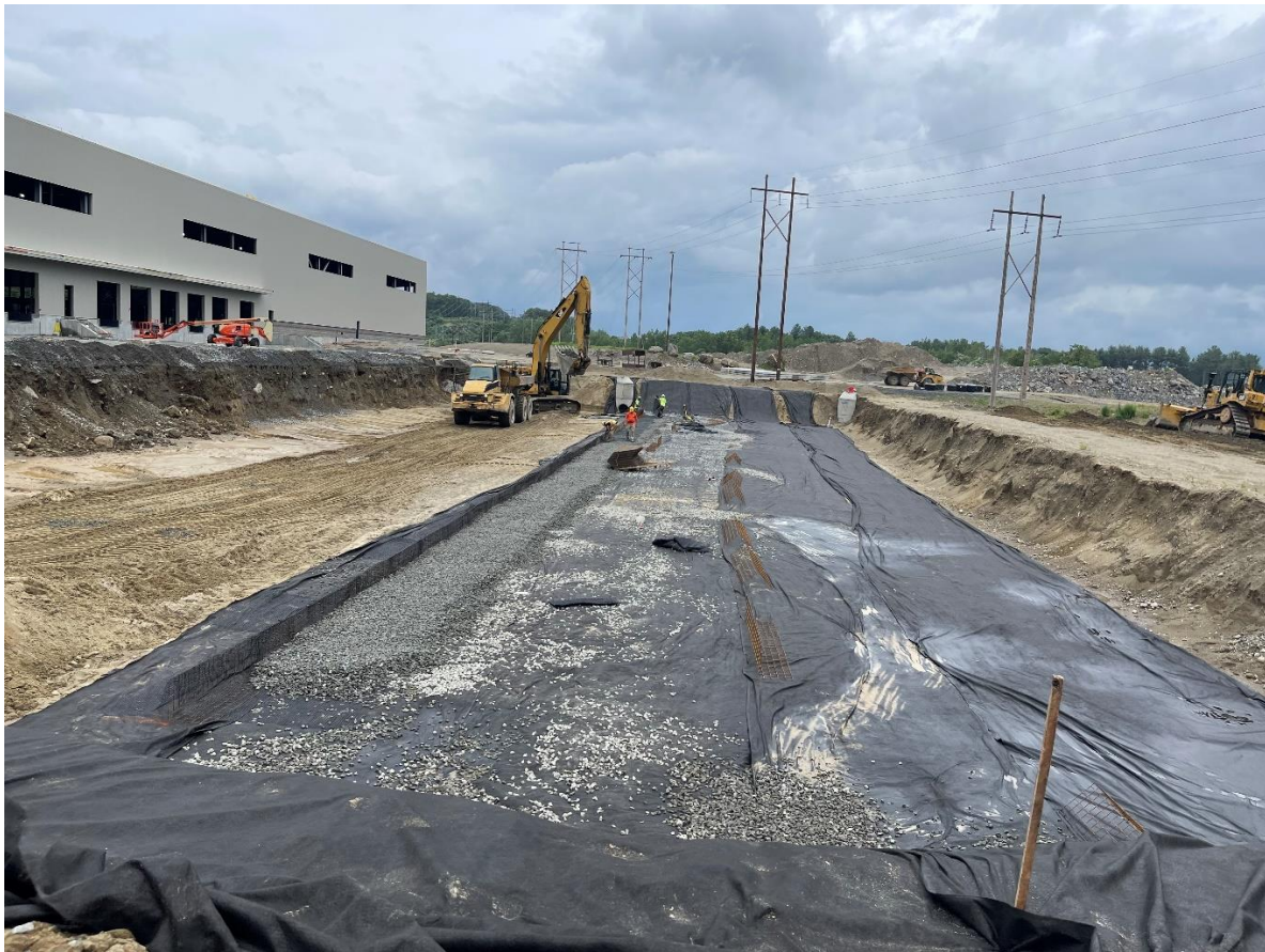
Photo 1: Geotextile fabric was placed along the bottom, northern, and southern sides of the eastern portion of SWMA UG3c.
