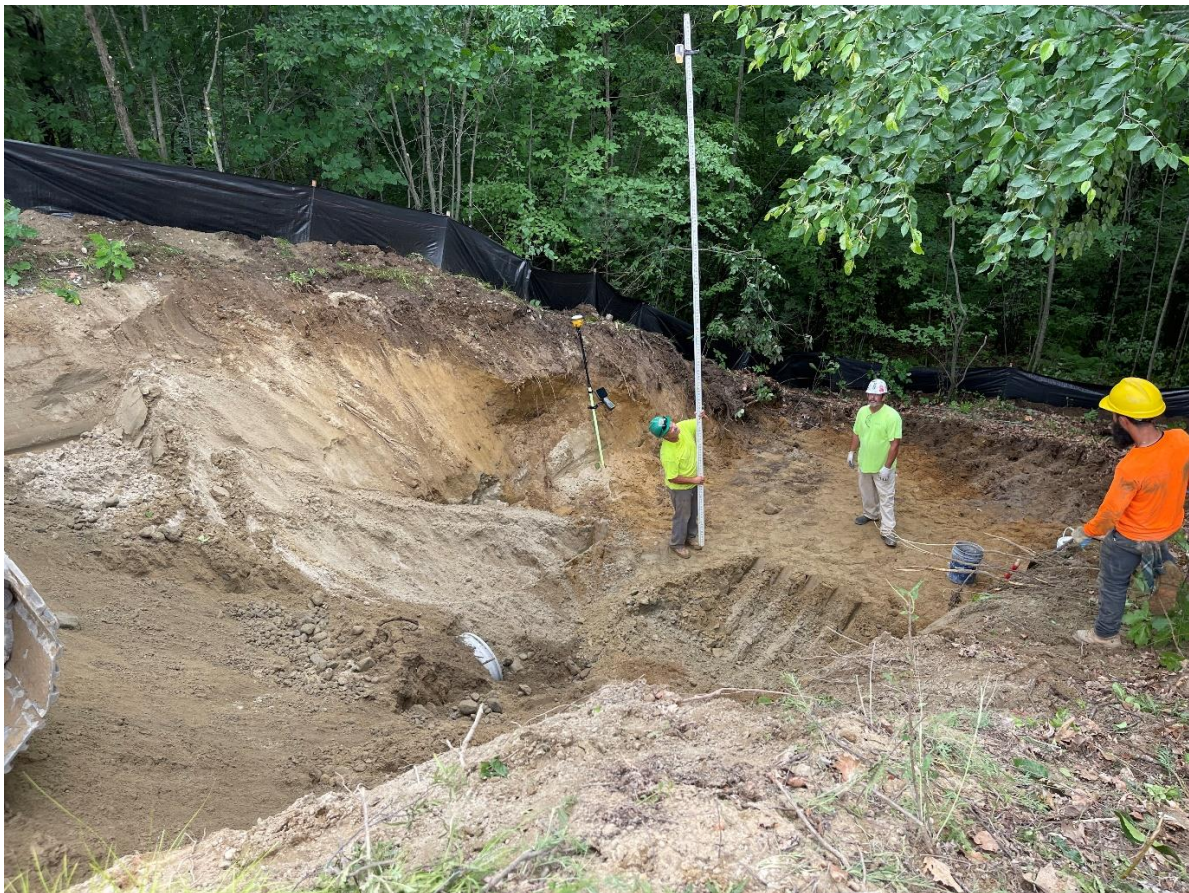
Photo 3: The contractor confirming elevations adjacent to the end of the pipe past DMH 506.
