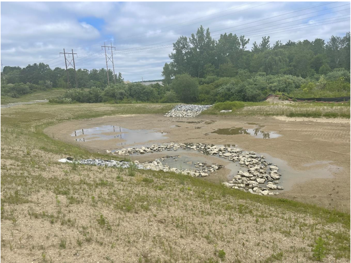
Photo 2: SWMA #3 was experiencing approximately 50% grass growth along the slopes, and no grass growth on the bottom.
