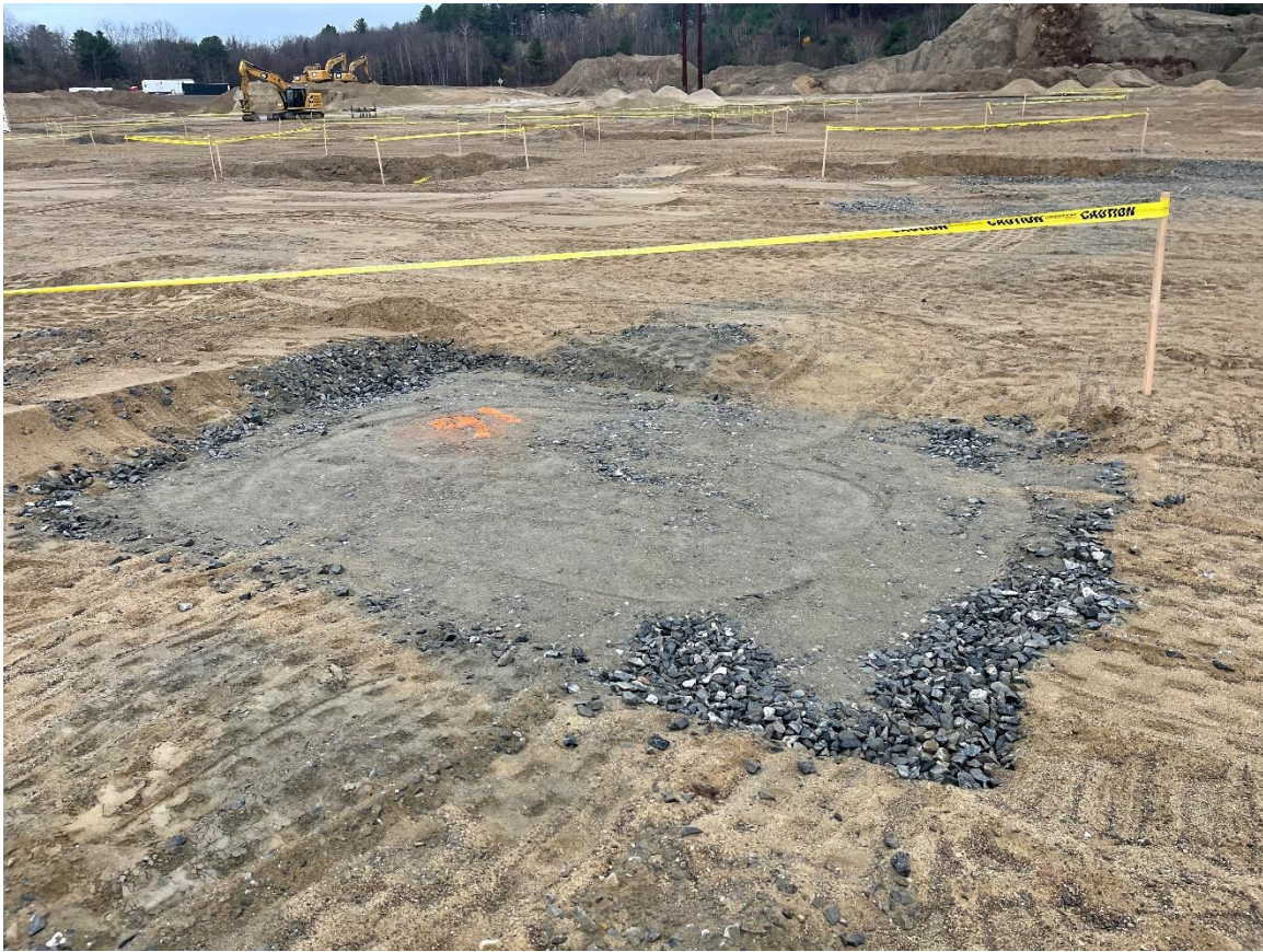
Photo 1: Gravel pads for what appears to be the columns of Building 3.
