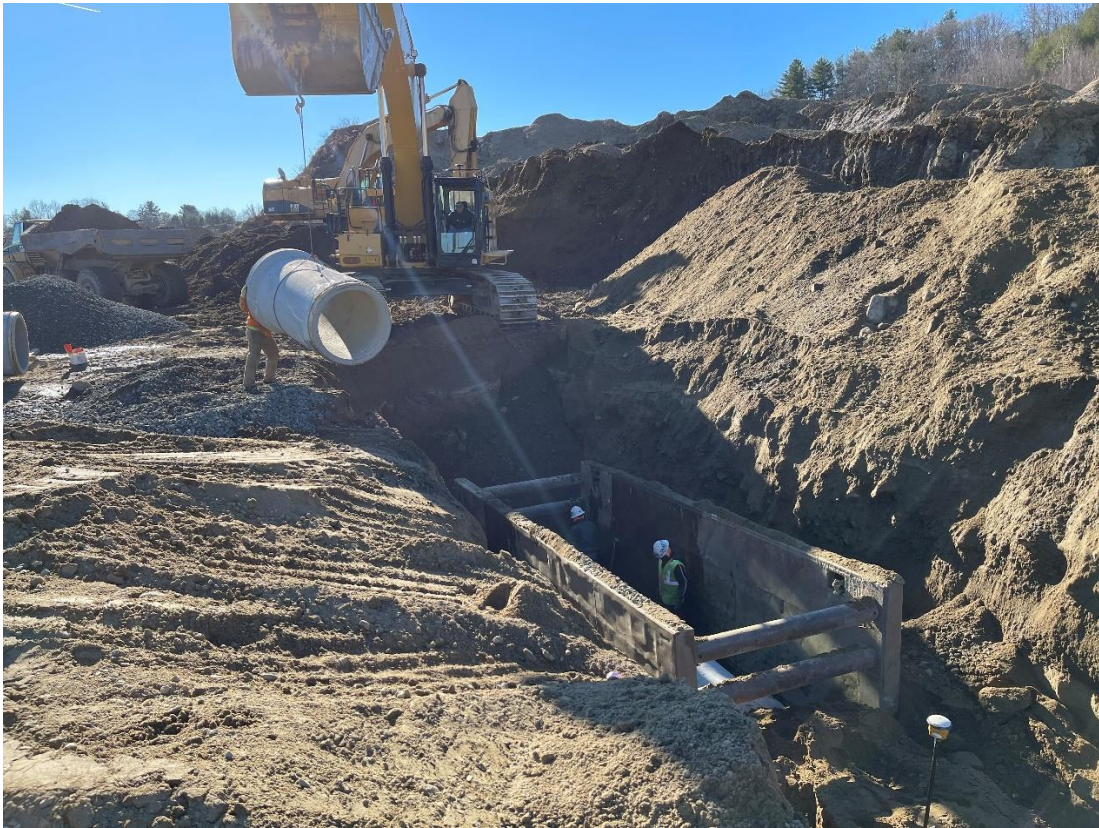
Photo 1: The contractor installed 16 feet of 36-inch RCP between DMH 604 and DMH 603.
