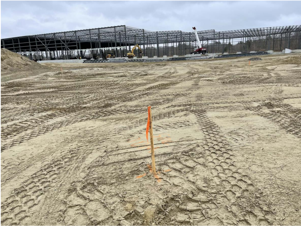
Photo 1: The locations of drainage structures had been staked throughout the site (WQU 705 shown).
