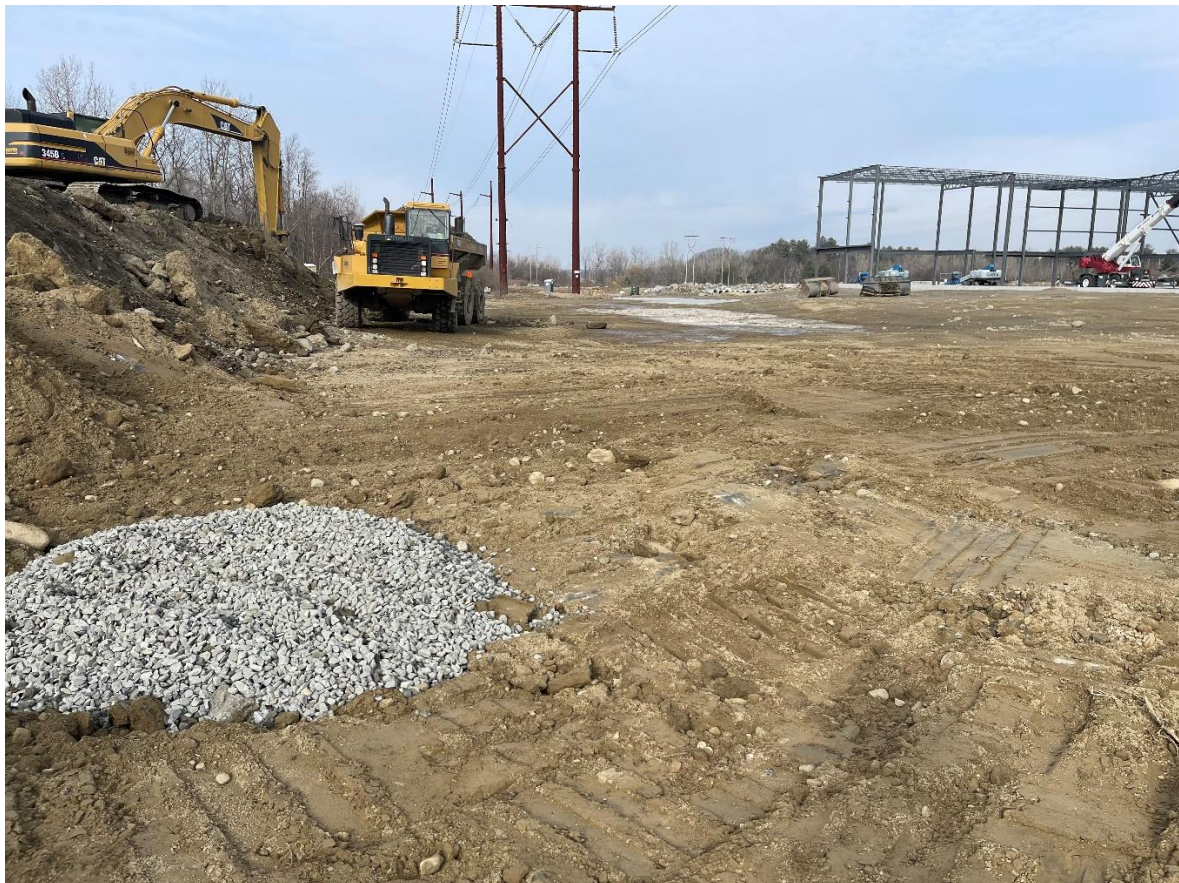
Photo 2: The 36-inch RCP between DMH 604 and DMH 603 had been backfilled, and DMH 603 covered in three-quarter-inch crushed stone.
