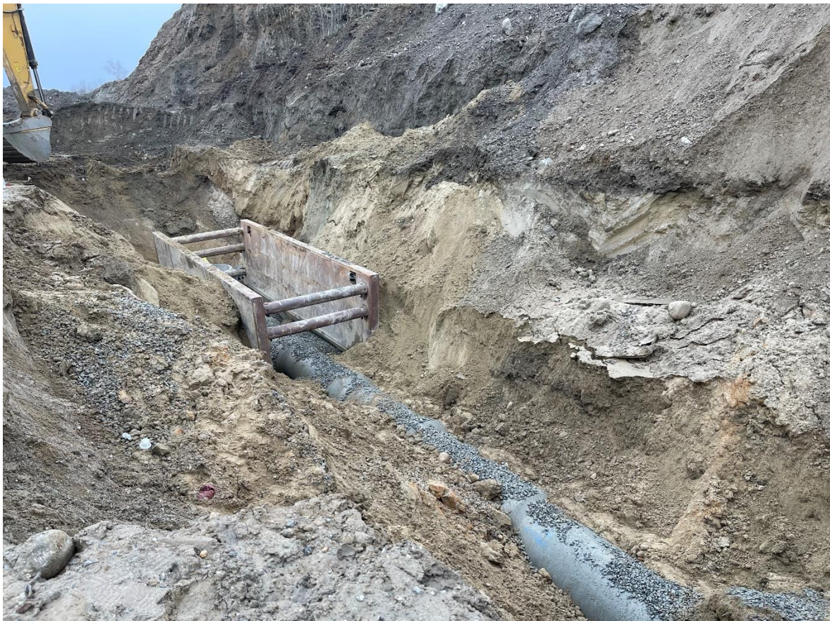
Photo 2: Approximately 80 feet of 24-inch RCP was installed and chinked between DMH 603 and DMH 601.
