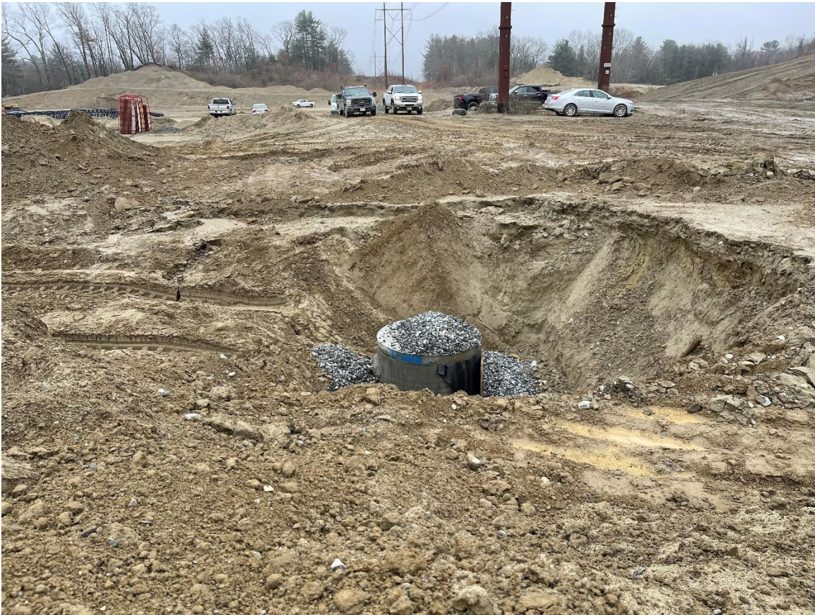
Photo 1: DMH 602 had been installed.
