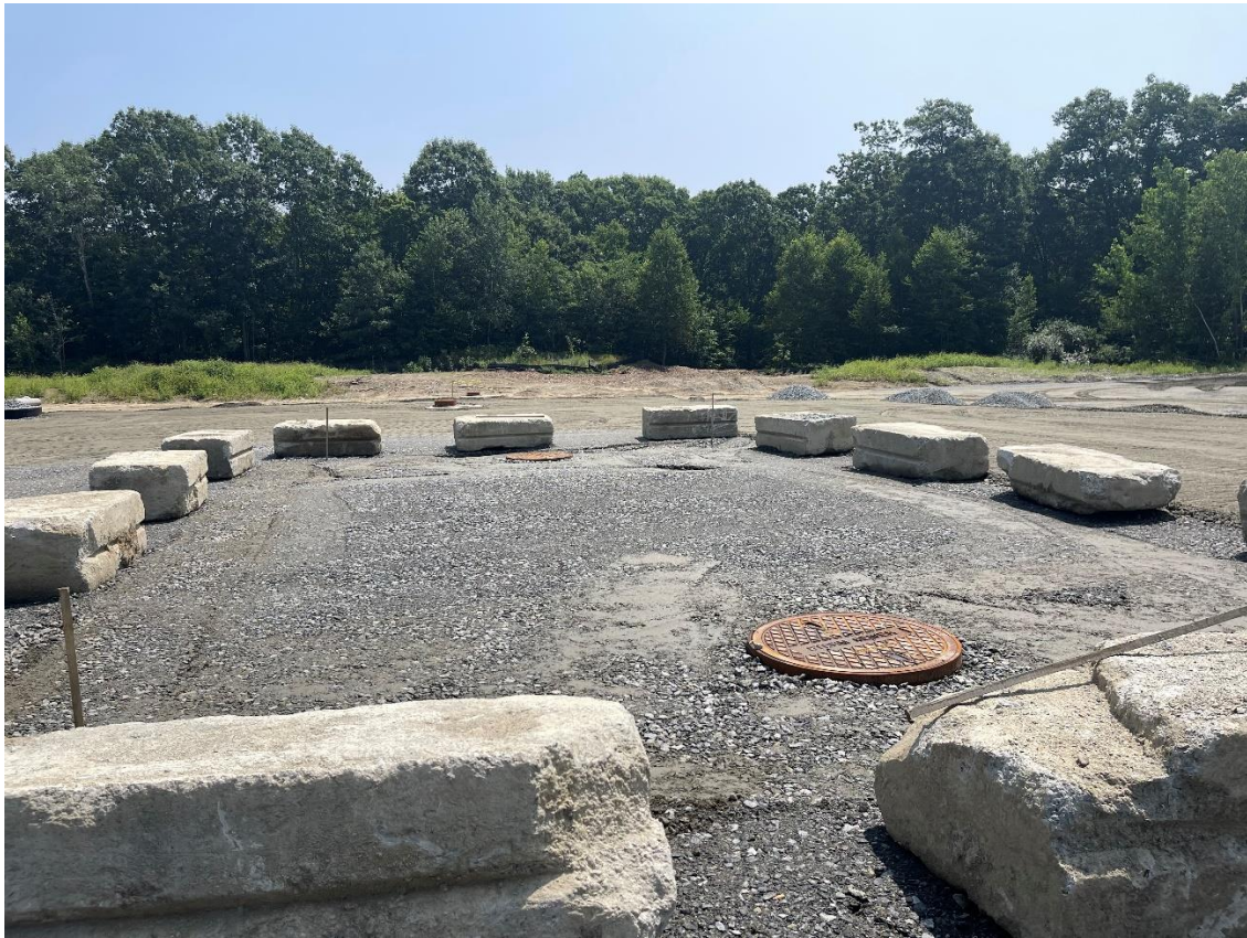
Photo 5: SWMA UG2e was covered in compacted dense-graded crushed stone. Two access manholes had been installed.
