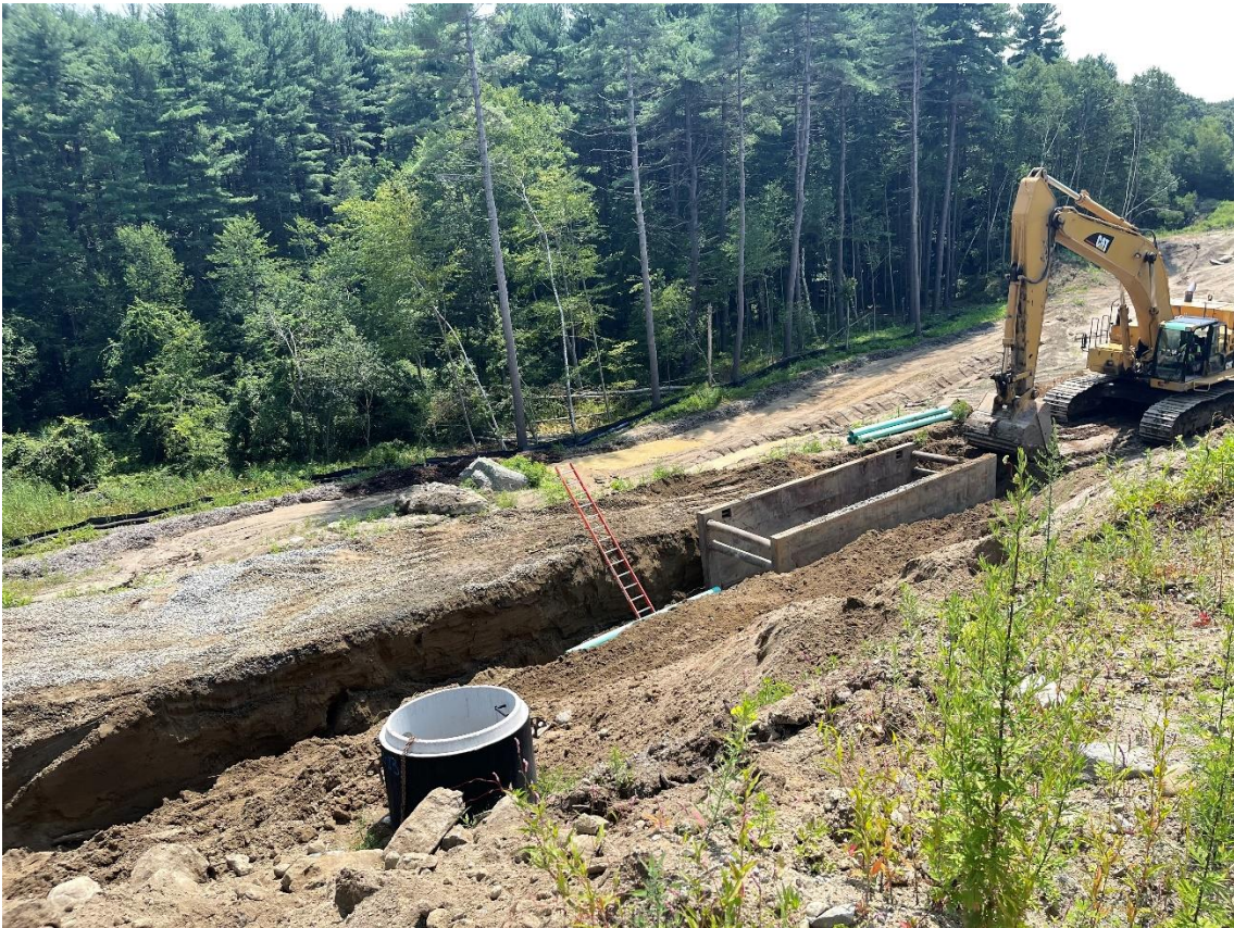
Photo 3: The contractor excavating the trench beyond the end of the pipe extending from SMH 107.
