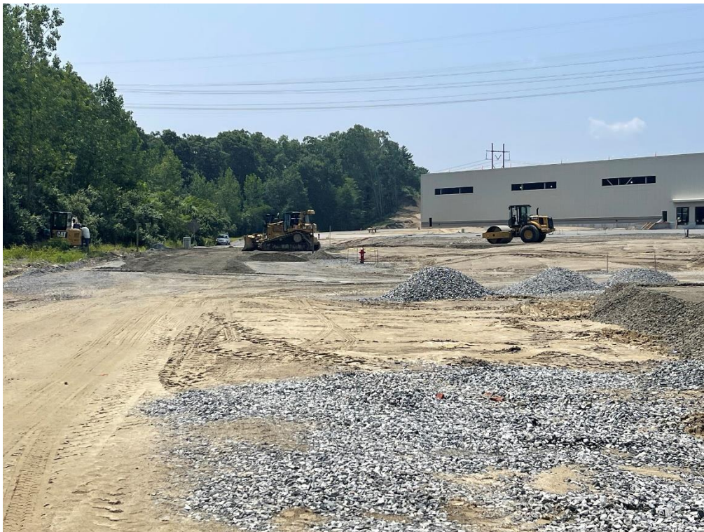
Photo 2: The contractor placing and compacting dense-graded crushed stone.
