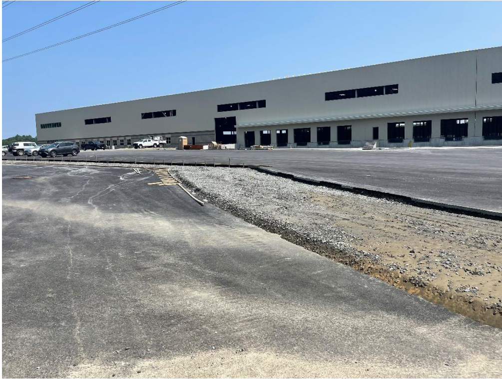
Photo 1: The areas for the concrete pads in the northern portion of the western lot had been prepared.
