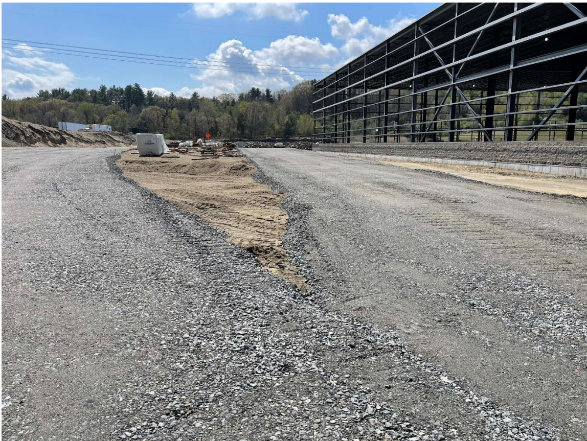
Photo 2: Dense-graded crushed stone had been placed and compacted along the main driveway as well as the driveway adjacent to the building along the southern side of Building 3.
