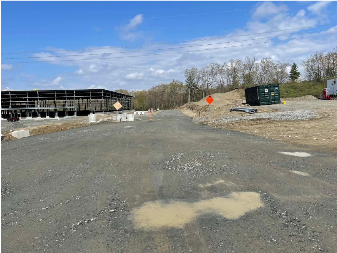
Photo 1: Dense-graded crushed stone had been placed and compacted along the southern driveway into Lot 3.
