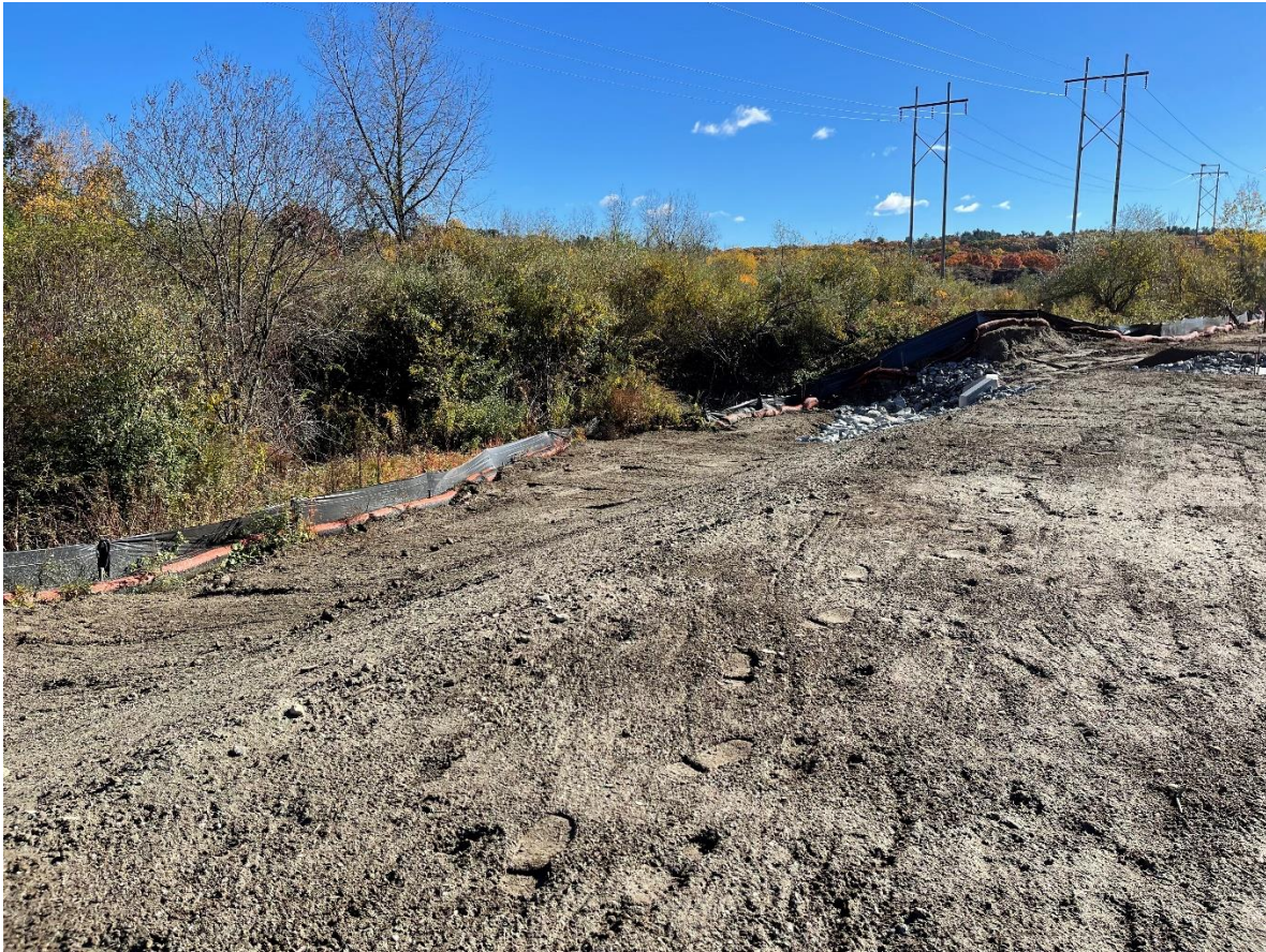
Photo 3: At SWMA #3, the topsoil at the outer slope near the emergency spillway had been repalced to avoid water pooling.
