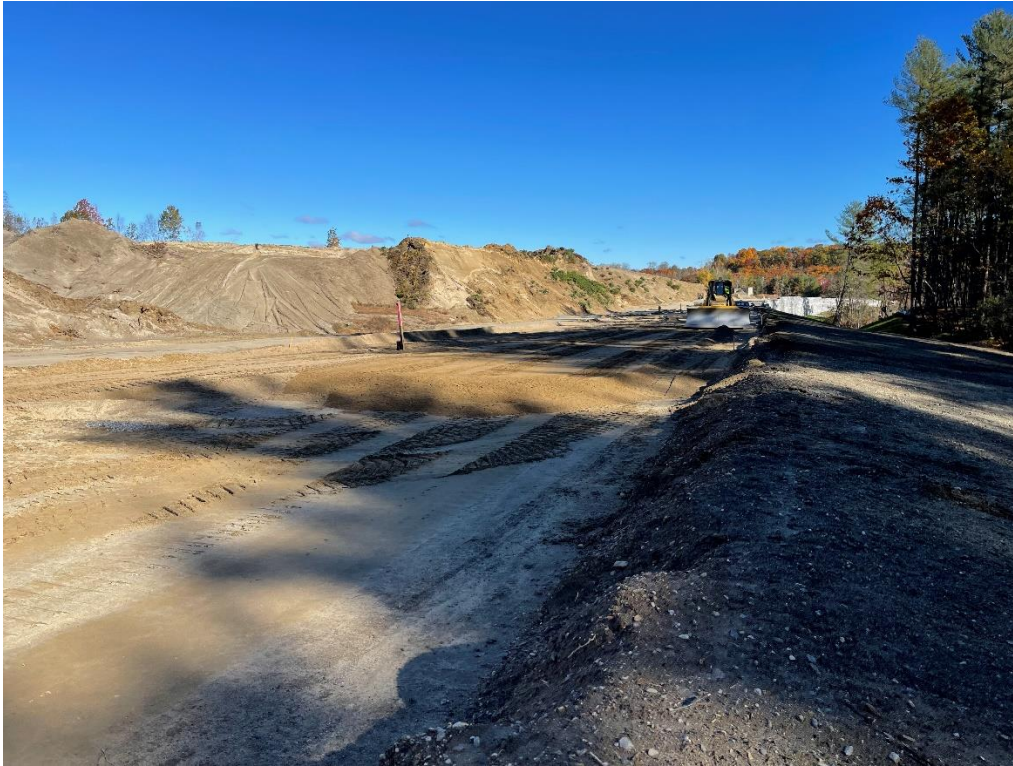
Photo 1: Between stations 8+00 and 8+50 the contractor was spreading a one-foot lift of backfill material across the right-of-way.
