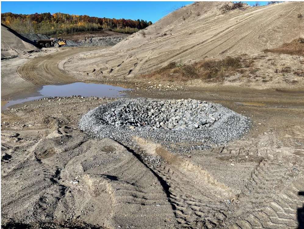
Photo 2: The riprap at FES 3A had been installed.
