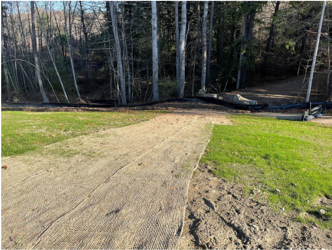
Photo 3: The area with jute matting between stations 8+00 and 9+00 was beginning to experience grass growth.
