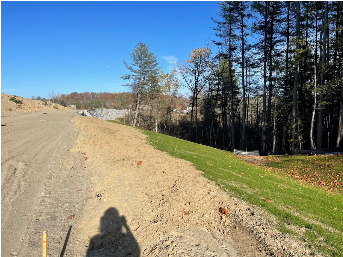
Photo 2: The uppermost portion of the slope between stations 8+00 and 9+00 needs to be reseeded.
