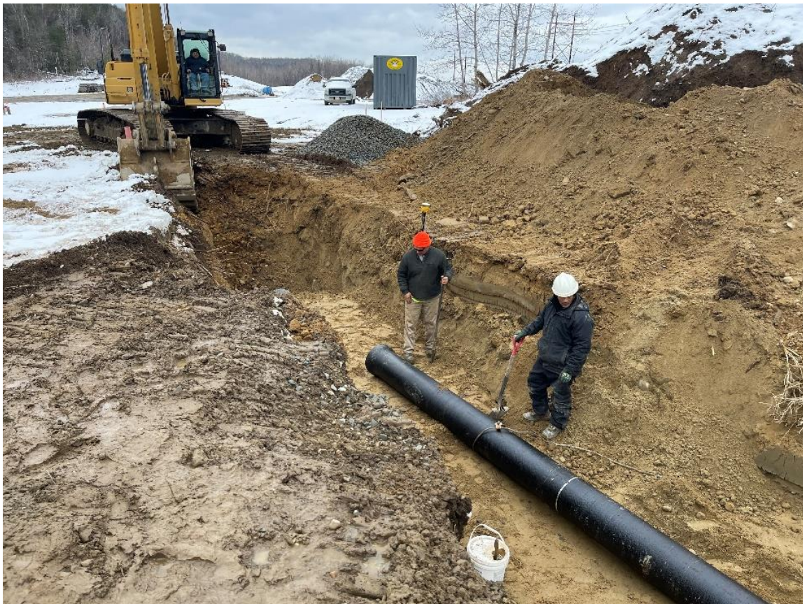
Photo 2: The contractor was excavating the pipe trench beyond the ends of the pipes.
