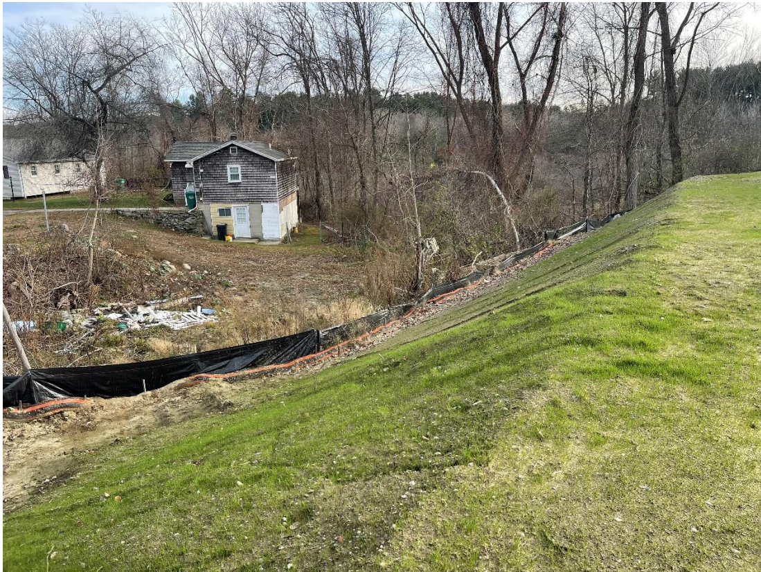
Photo 1: The silt fence between SWMA #1 and N/F Vaillancourt will need to be cleaned out.
