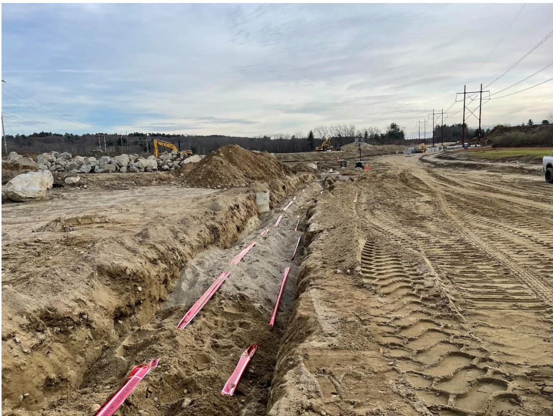
Photo 2: Electrical conduit installed between stations 31+00 and 34+00.
