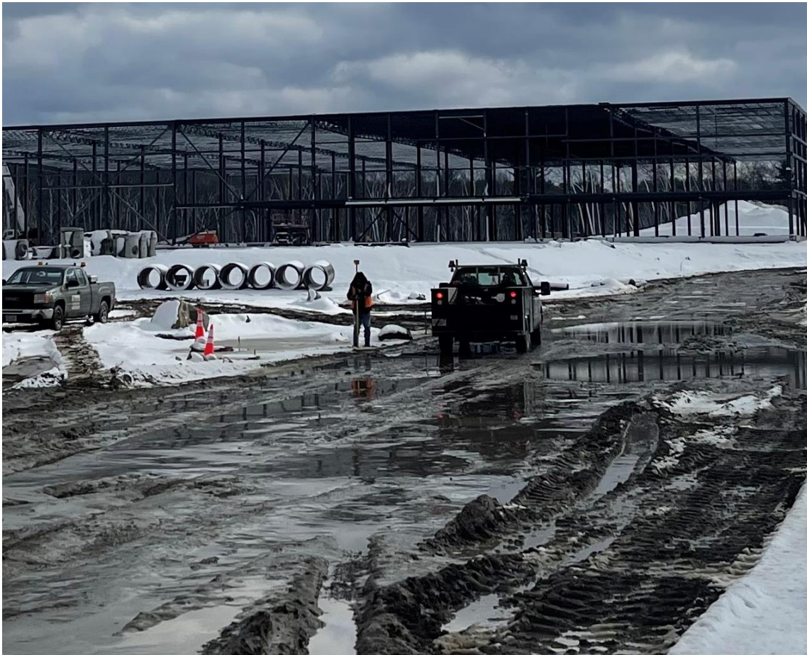
Photo 1: The contractor marking locations with a GPS.
