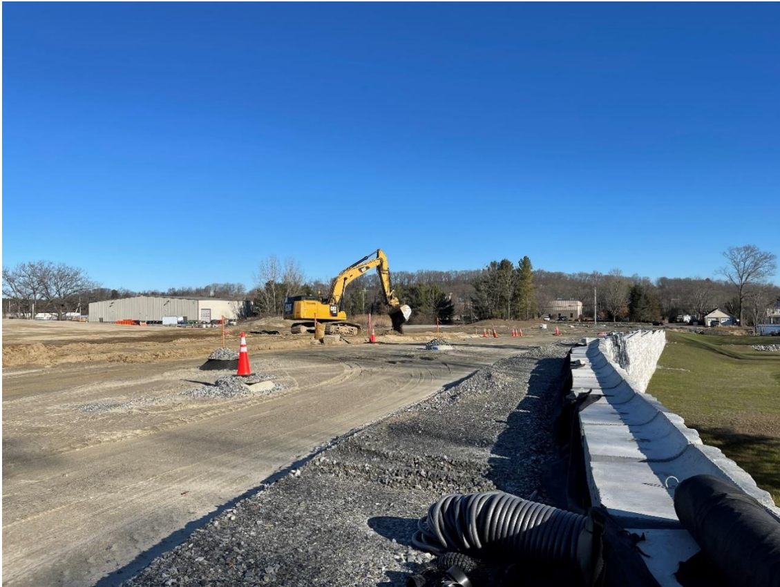
Photo 1: The contractor backfilling the electrical utilities as well as placing earth material outside the right-of-way.
