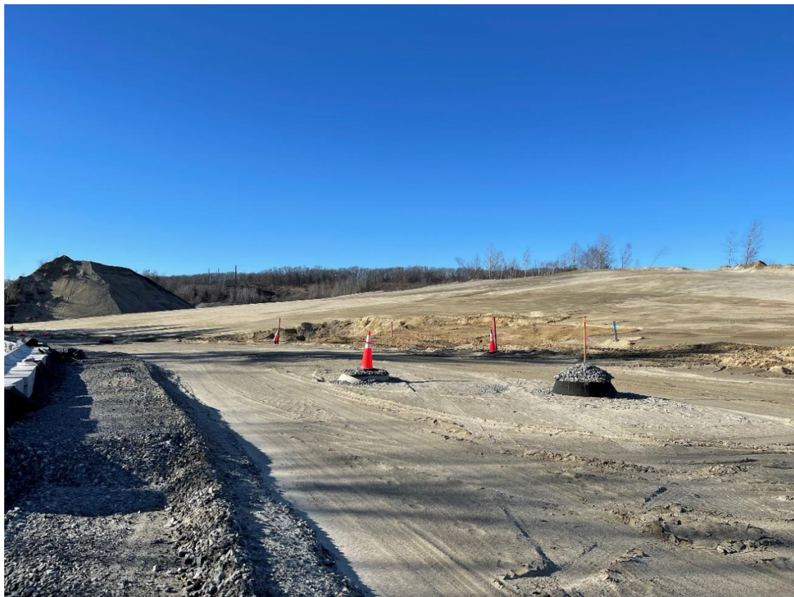
Photo 2: The slope outside the right-of-way between stations 5+00 and 7+00 had been graded.
