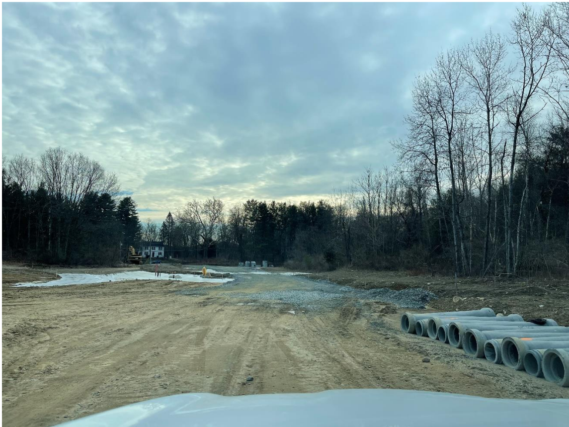
Photo 2: Three-quarter-inch crushed stone had been placed along the roadway between stations 52+00 and 56+00.
