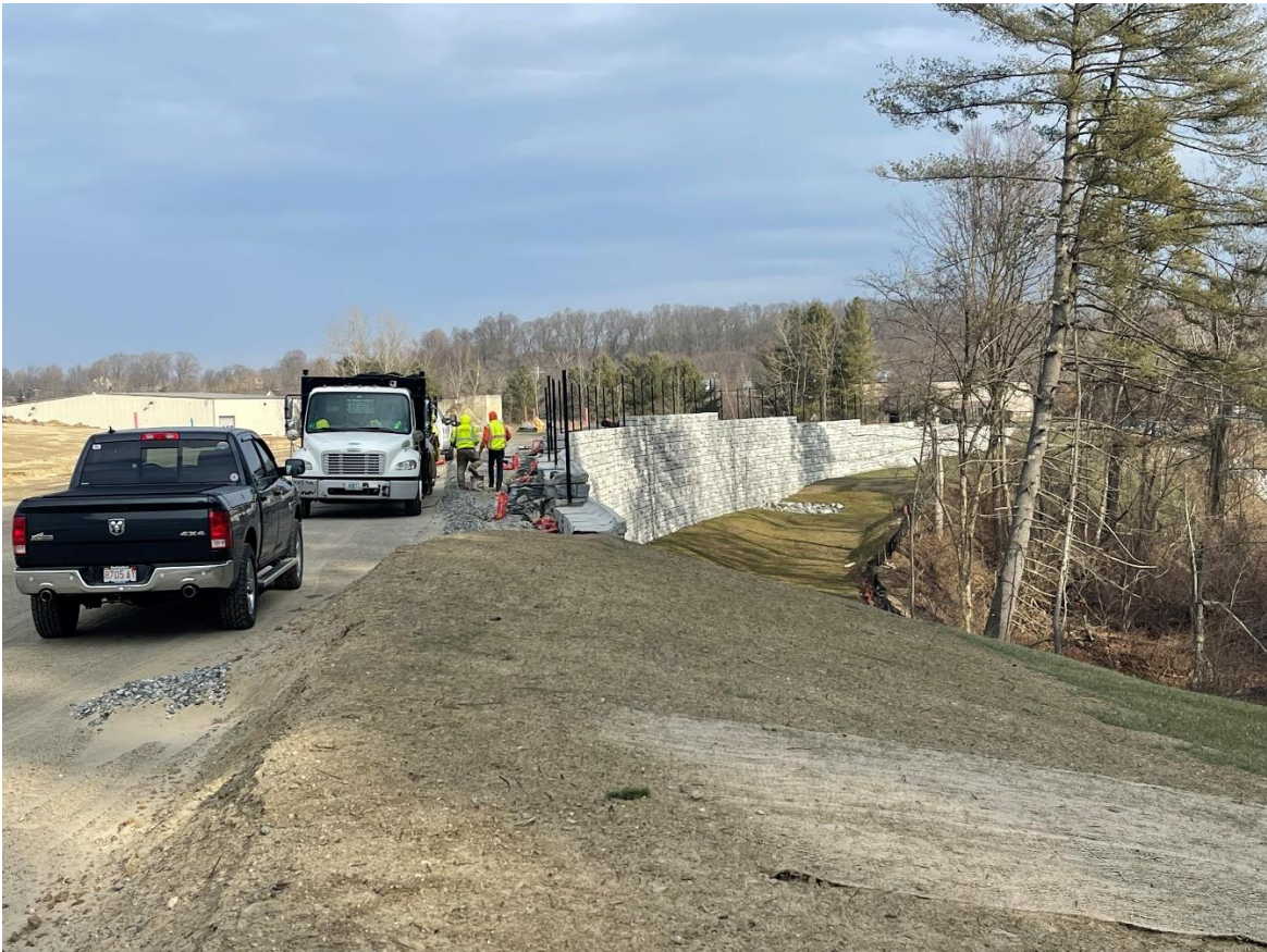
Photo 1: The contractor was installing the posts of the chain link fence along the retaining wall.
