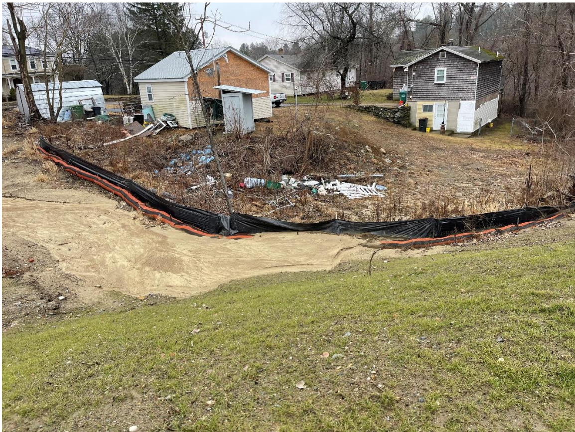
Photo 2: A significant amount of sediment had accumulated in the silt fence between the eastern corner of SWMA #1 and the property line.
