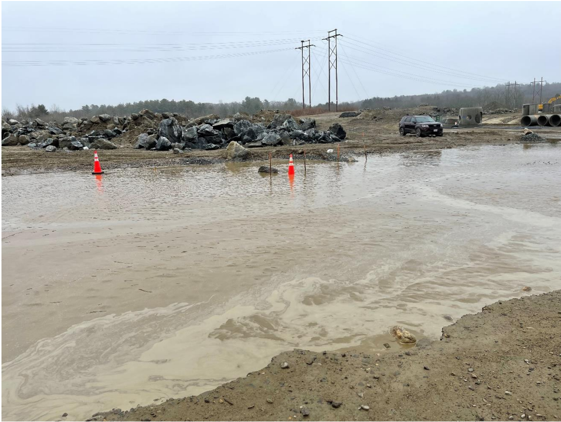
Photo 3: A significant amount of runoff had pooled at approximately station 38+00, at the intersection of the subdivision road and the driveway leading to Lots 2 and 3.
