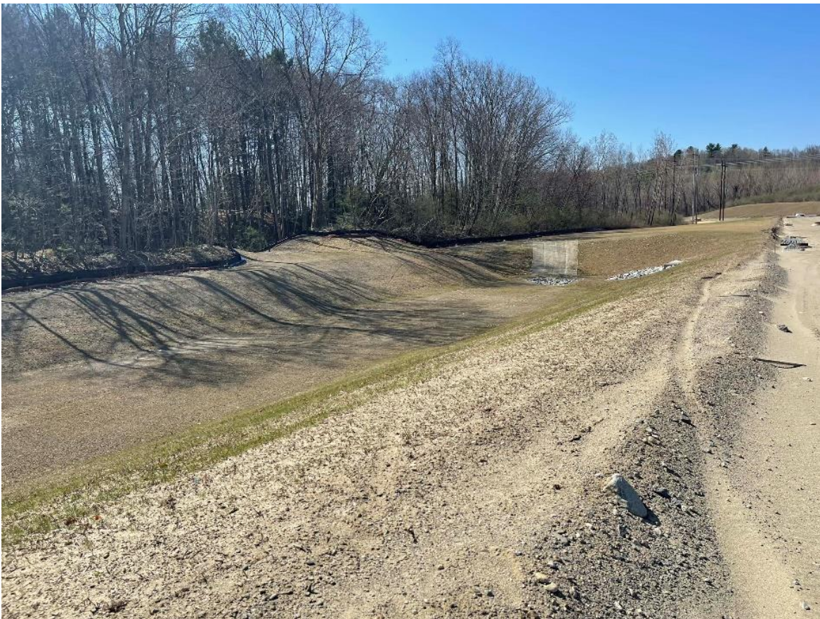
Photo 2: SWMA #2 was experiencing sparse grass growth, and the jute matting in the northern corner was in good condition.
