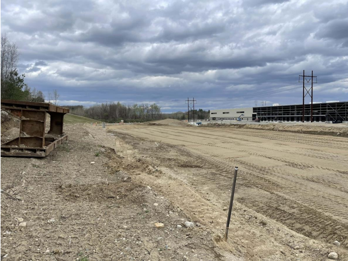
Photo 1: The right-of-way between stations 47+00 and 50+00 had been brought to subgrade.
