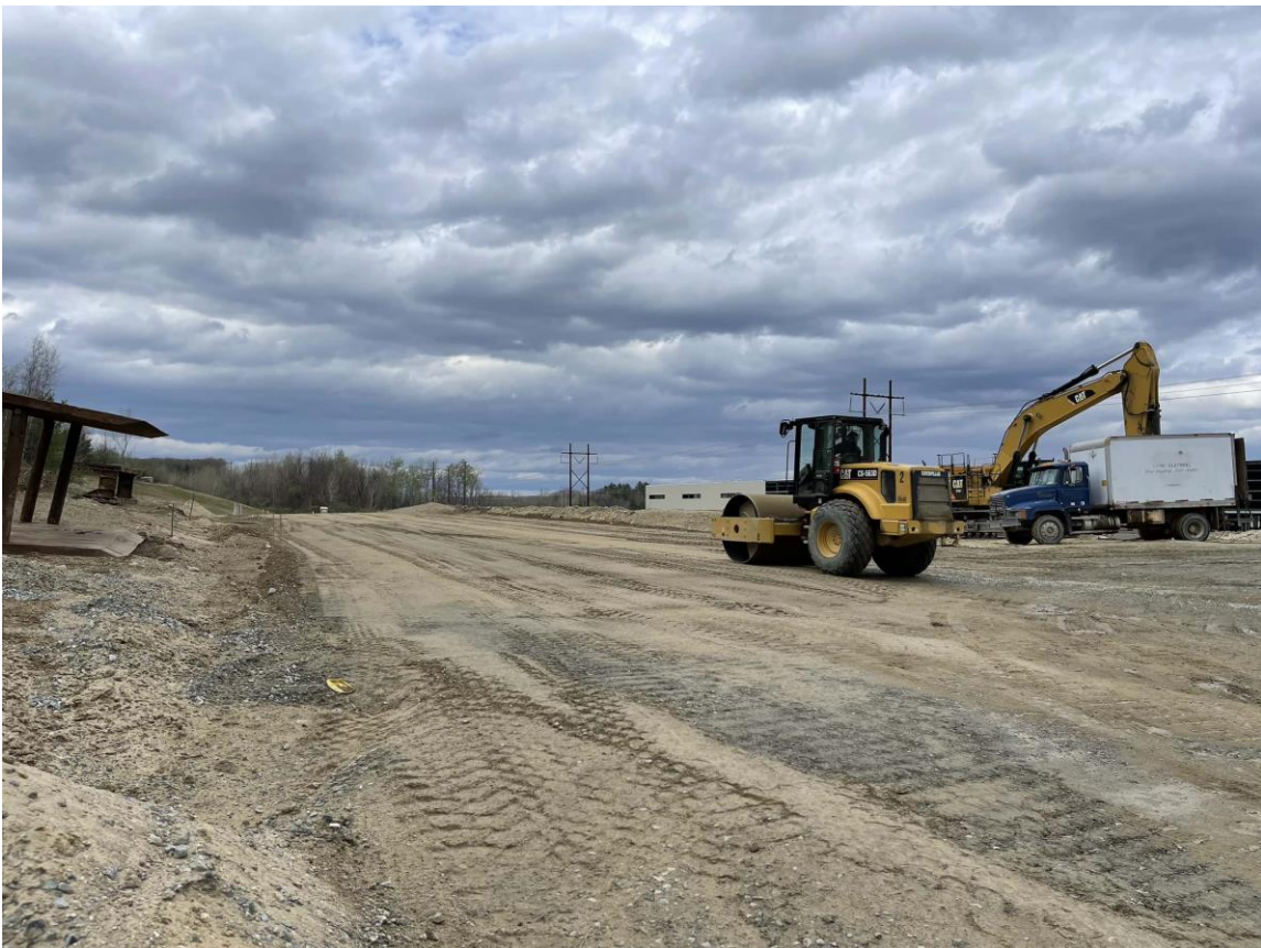
Photo 2: The contractor was compacting the right-of-way with a 10-ton roller.
