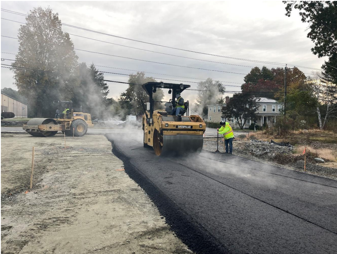
Photo 1: The contractor compacting asphalt at approximately station 0+50.
