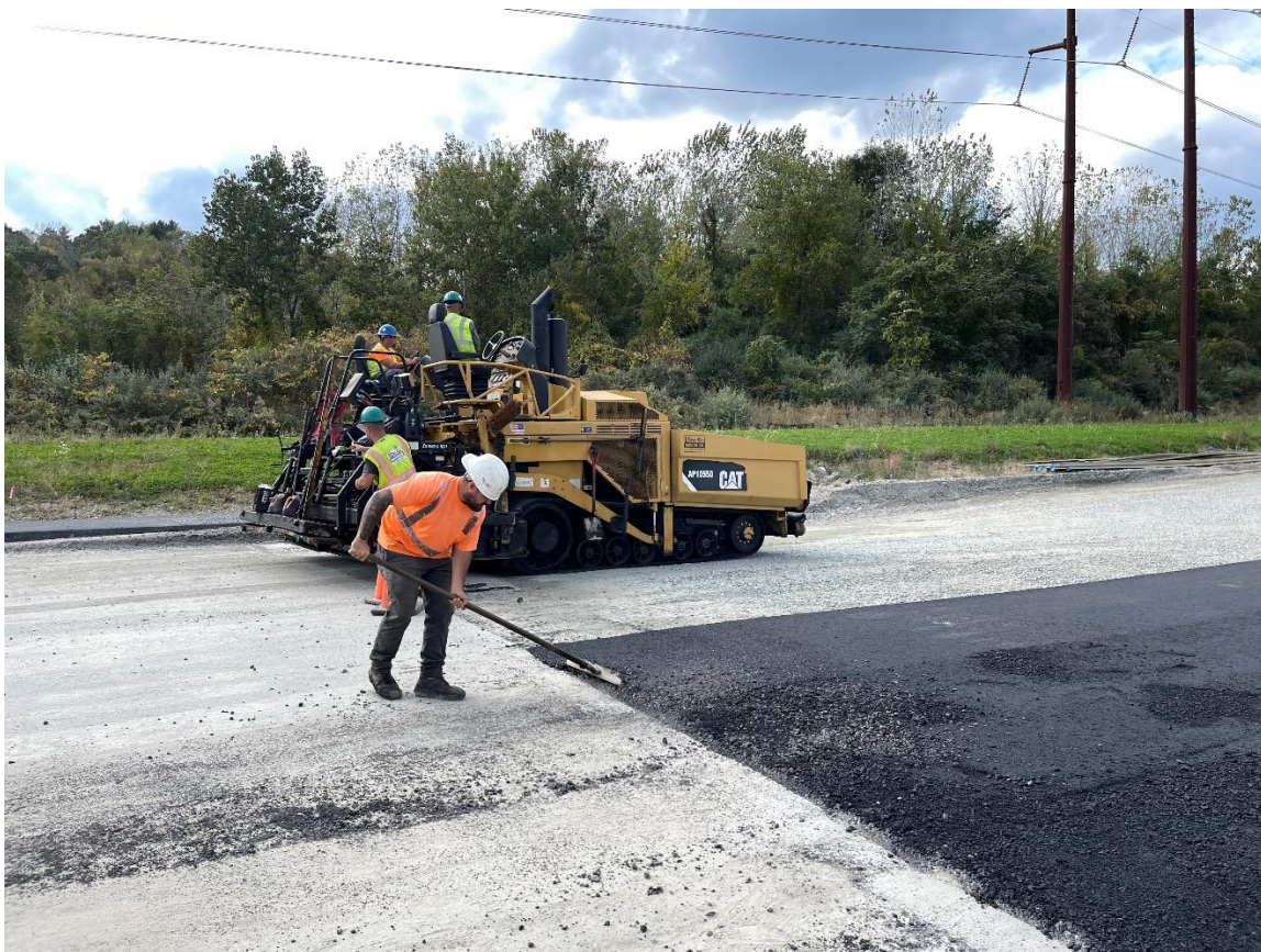
Photo 2: The contractor placing asphalt at station 35+50.
