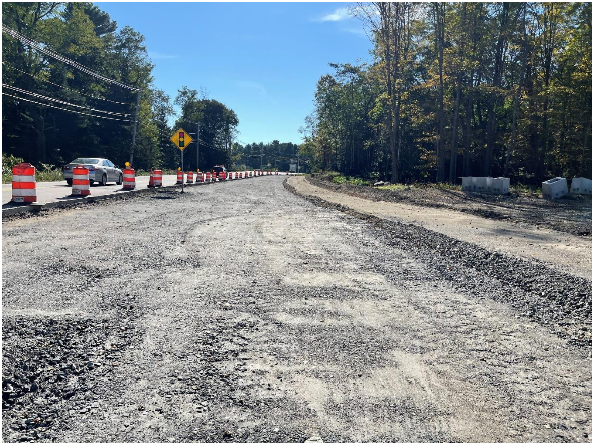
Photo 7: The dense graded crushed stone in the Boston Road modification areas had been fine graded.
