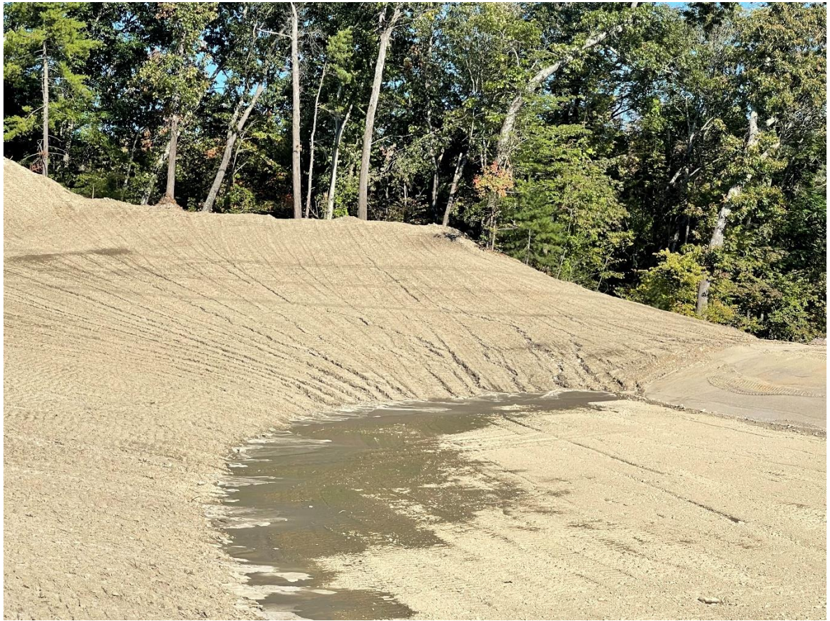
Photo 6: Erosion rills had formed along the eastern slope of SWMA #4.
