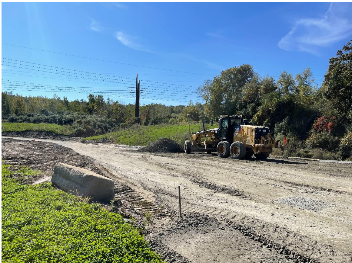
Photo 5: The contractor was fine grading at station 22+00.
