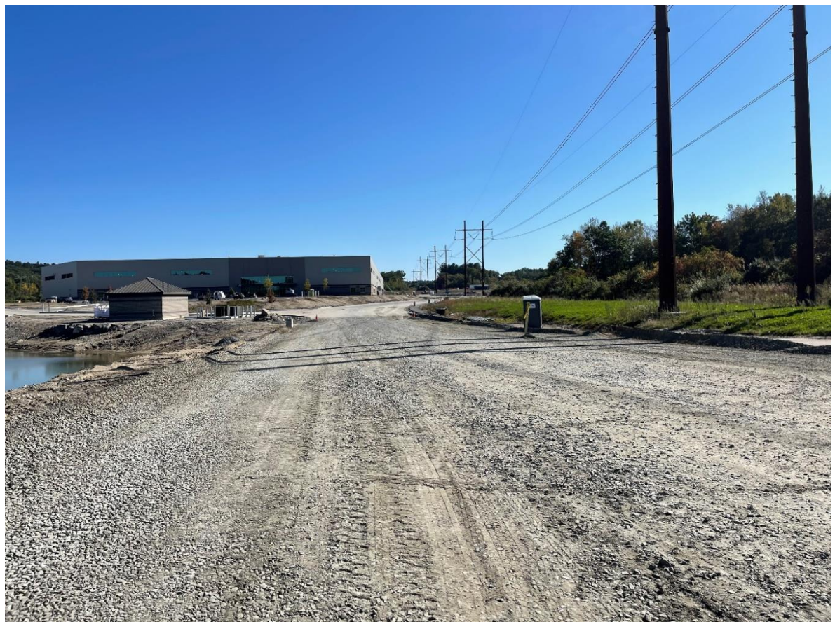
Photo 3: General conditions of the dense graded crushed stone at approximately station 32+00 facing towards 56+00.
