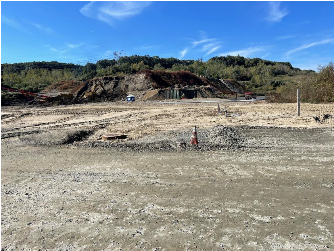
Photo 4: The area immediately surrounding the electrical manhole did not have dense graded crushed stone.
