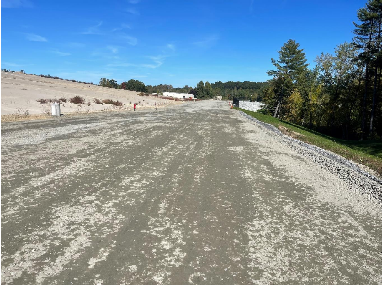
Photo 1: General conditions of the dense graded crushed stone at approximately station 19+00 facing towards 0+00.
