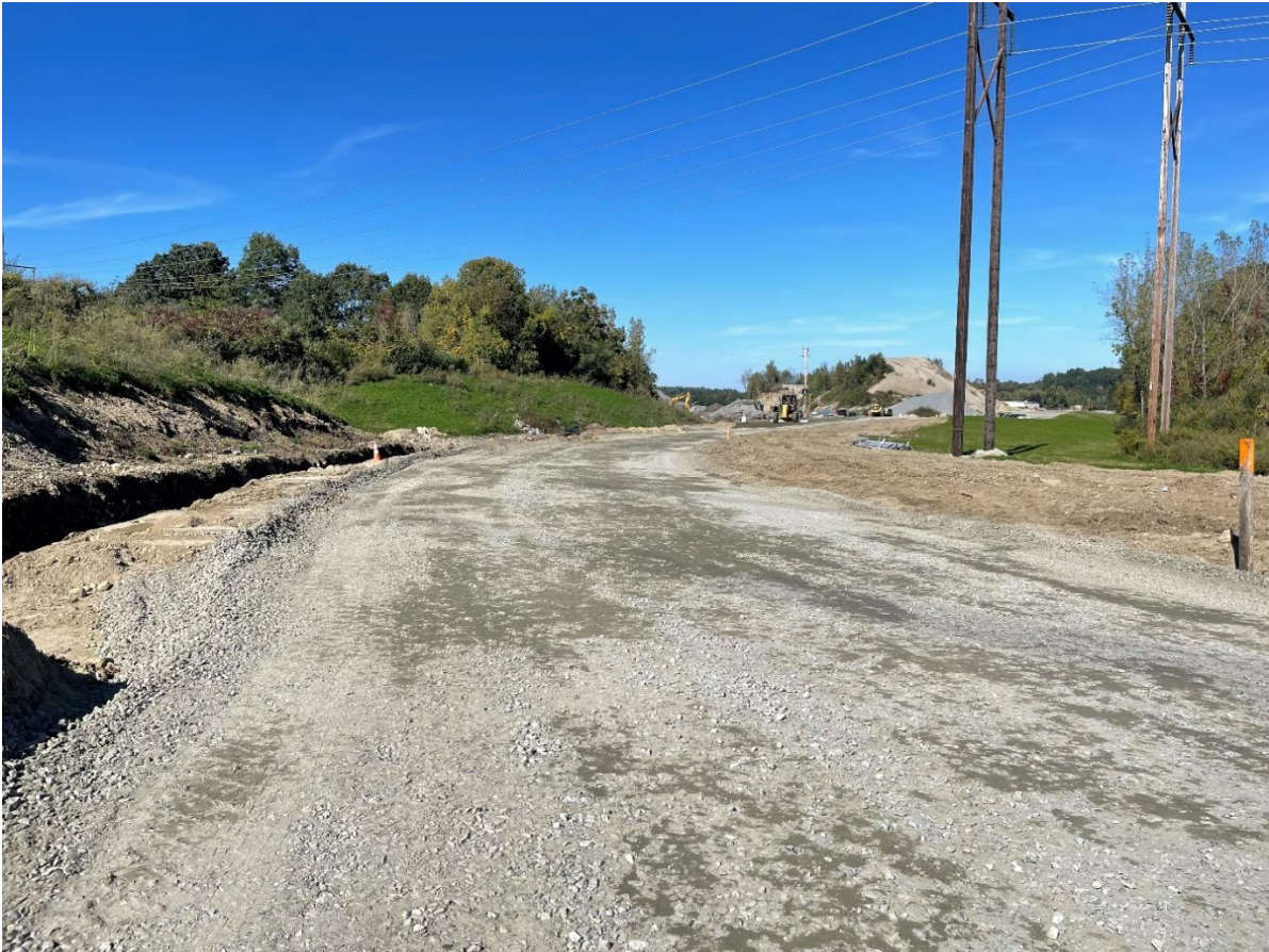
Photo 2: General conditions of the dense grade crushed stone at approximately station 26+00 facing towards 0+00.
