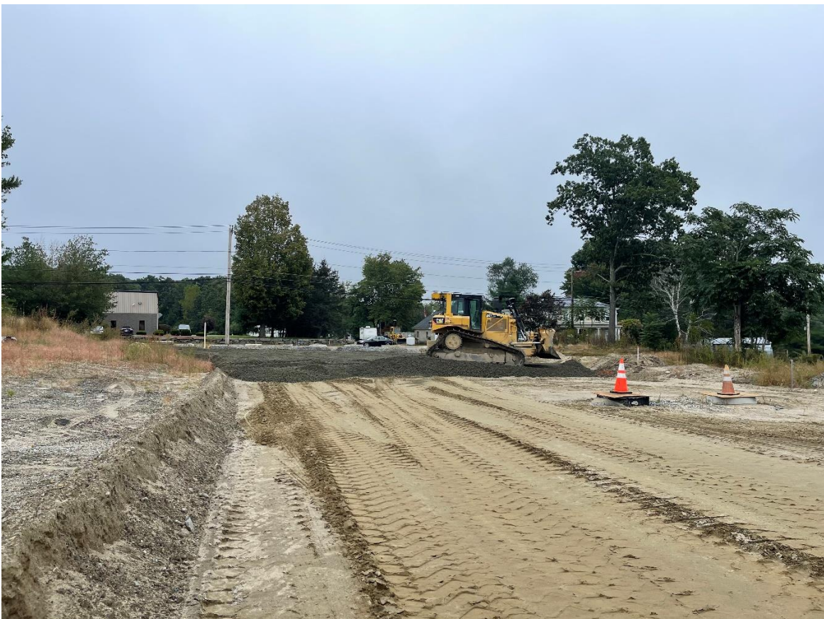
Photo 4: The contractor placing dense grade crushed stone at station 0+90.
