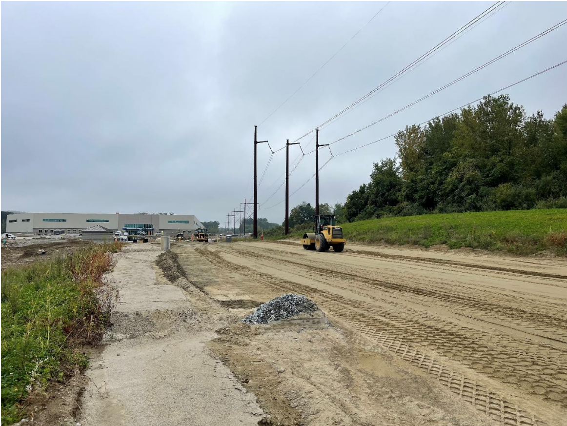
Photo 3: The contractor compacting the roadway between stations 30+00 and 32+00.
