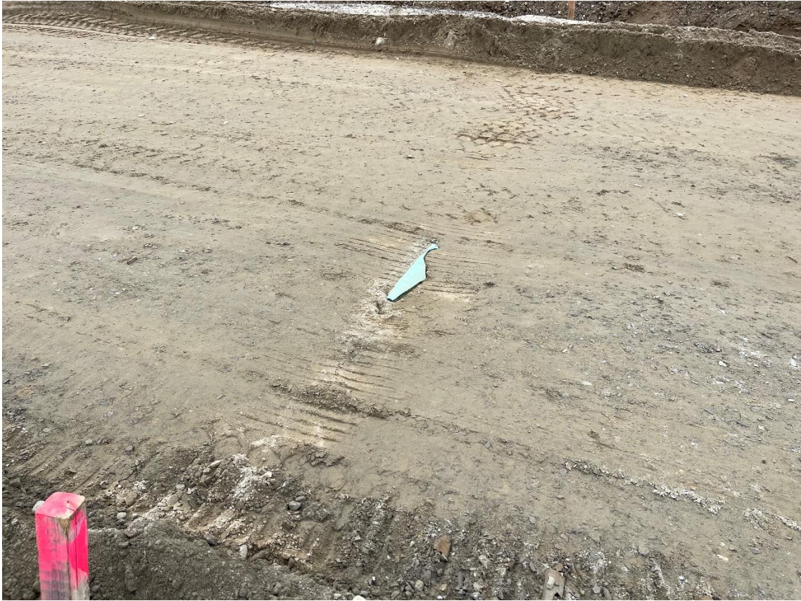
Photo 5: The exposed portion of the SDR pipe at station 27+00 was broken.
