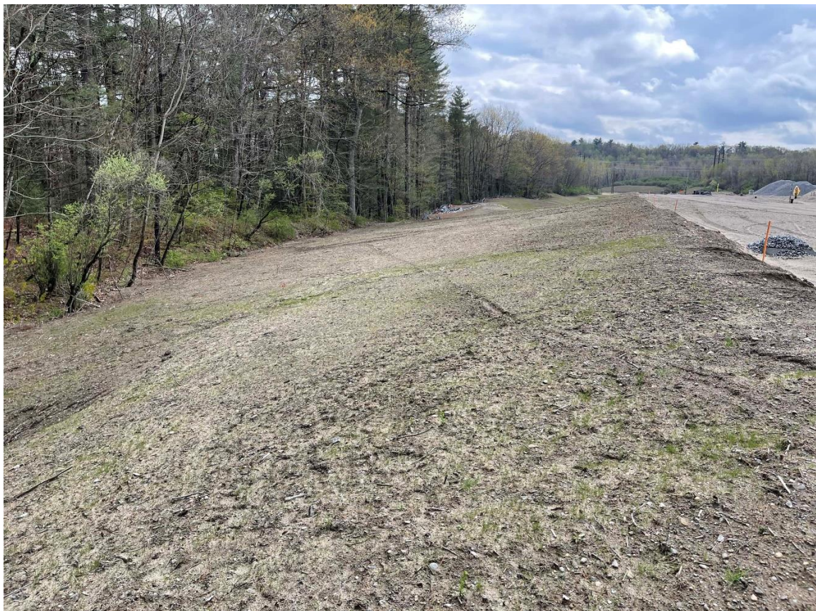
Photos 1 and 2: Areas experiencing less than 70% grass coverage (SWMA #1 and the slope between the retaining wall and SWMA #2 shown) may have to be reseeded to encourage additional grass growth.
