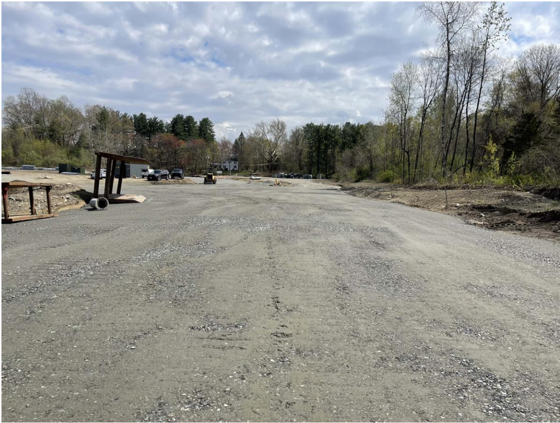
Photo 3: Dense-graded crushed stone had been placed and compacted along the right-of-way between stations 50+00 and 56+00 to a width of 50 feet.
