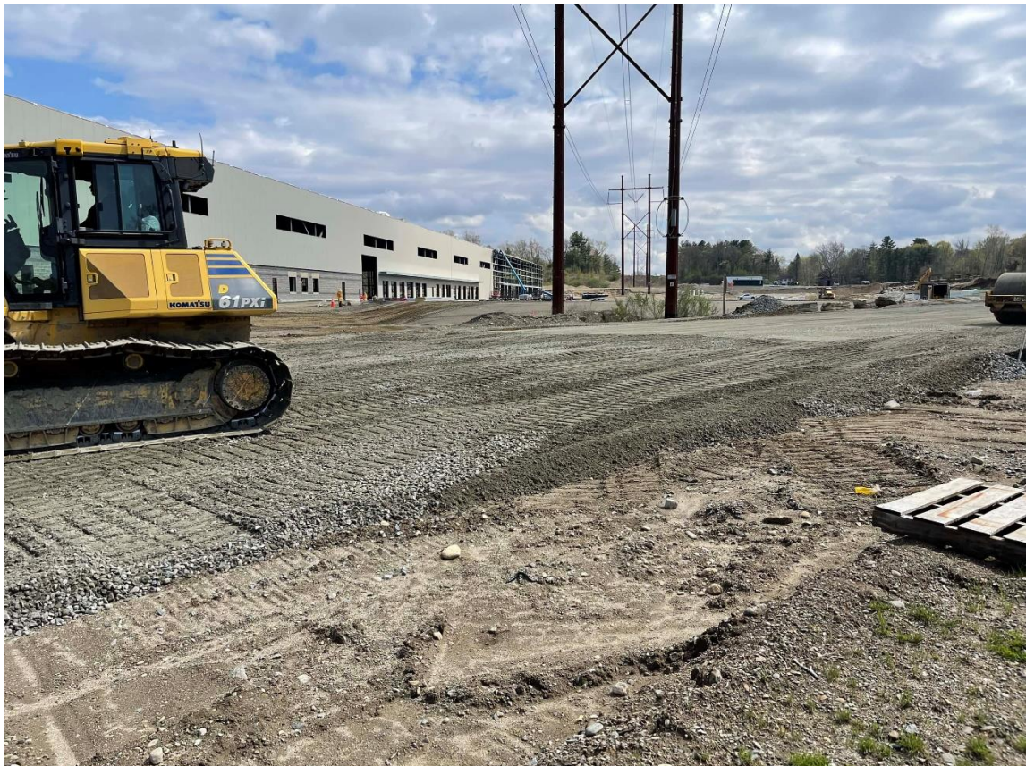
Photo 4: The contractor placing a one-foot lift of dense-graded crushed stone at approximately station 39+00.
