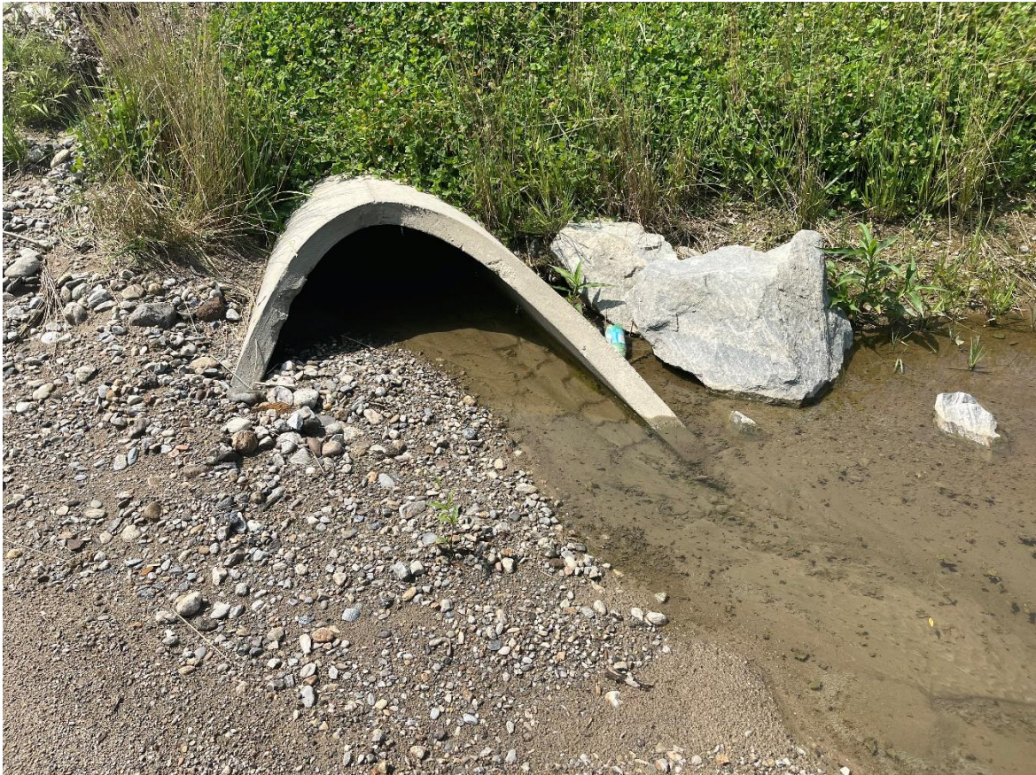
Photo 1: Sediment had accumulated in FES-301 and needs to be cleaned out.
