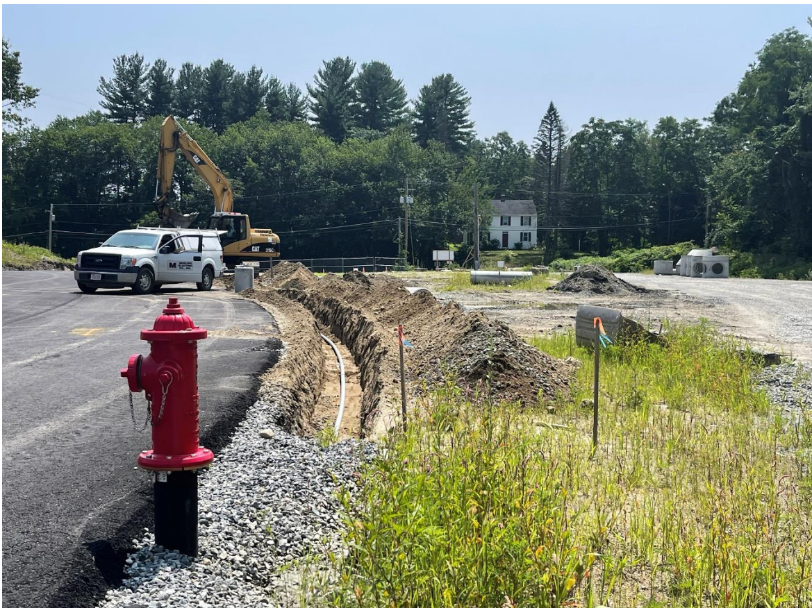
Photo 3: The contractor installing electrical conduit pipe at approximately station 52+50.
