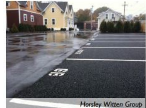
This parking lot in Narragansett, RI shows traditional asphalt on the left, where puddles have formed, and permeable pavement on the right, where it has soaked through.
