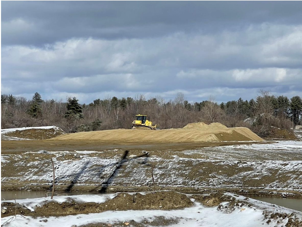
Photo 1: The contractor placing earth material at the location of the southern parking lot/southern side of Building 2.
