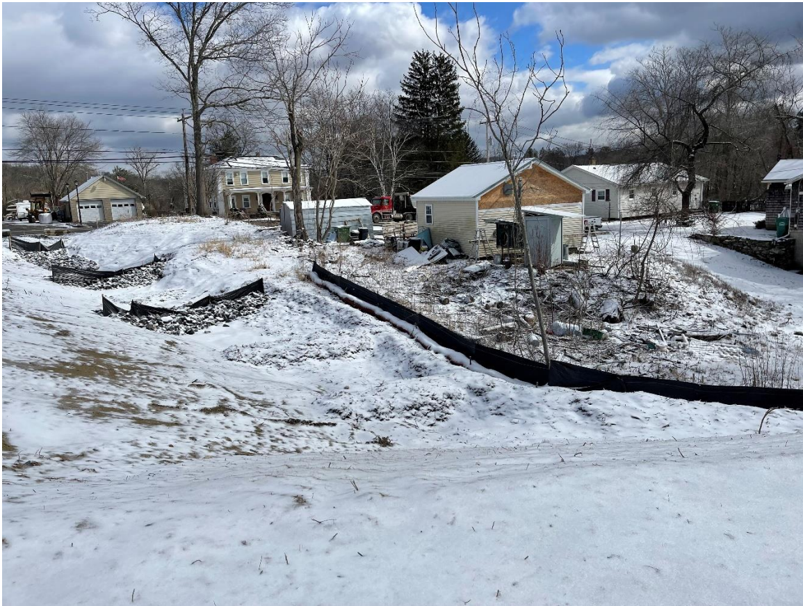
Photo 1: The silt fence and stump grindings between the eastern corner of Stormwater Management Area (SWMA) #1 and the property line were well-maintained.
