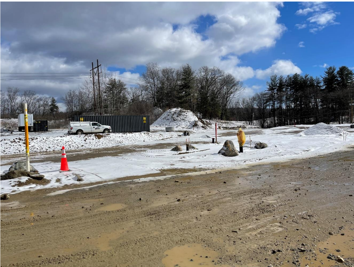
Photo 2: The previously installed gas utility pipe between stations 51+00 and 53+75 had been backfilled.
